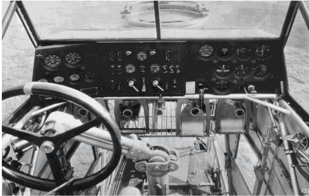
Figure 1. Keystone B-6A Cockpit without Attitude Indicator Source: The National Museum of the Air Force
