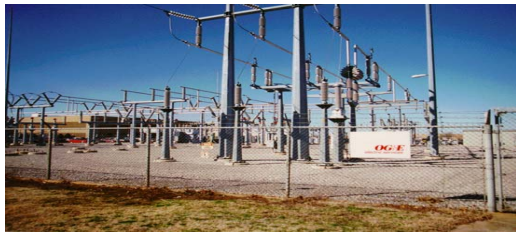
Sub Station A 12,470 Volt Feed
