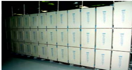
1200 Batteries/5000 kVA UPS
