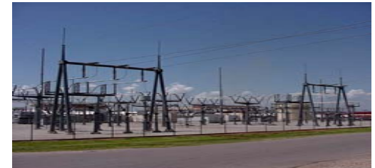
Sub Station B 12,470 Volt Feed
