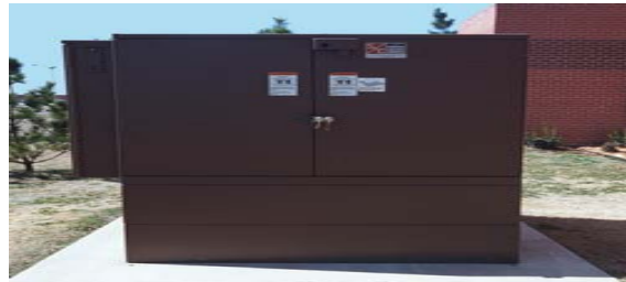
Automatic Transfer Switch
