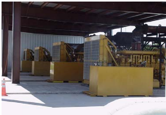
Four 1750 kW Diesel Generators
