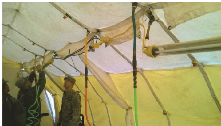
Figure 1. Soldiers setting up water and power lines in the Interior of a personnel decontamination tent. Figure courtesy of Massachusetts National Guard.
