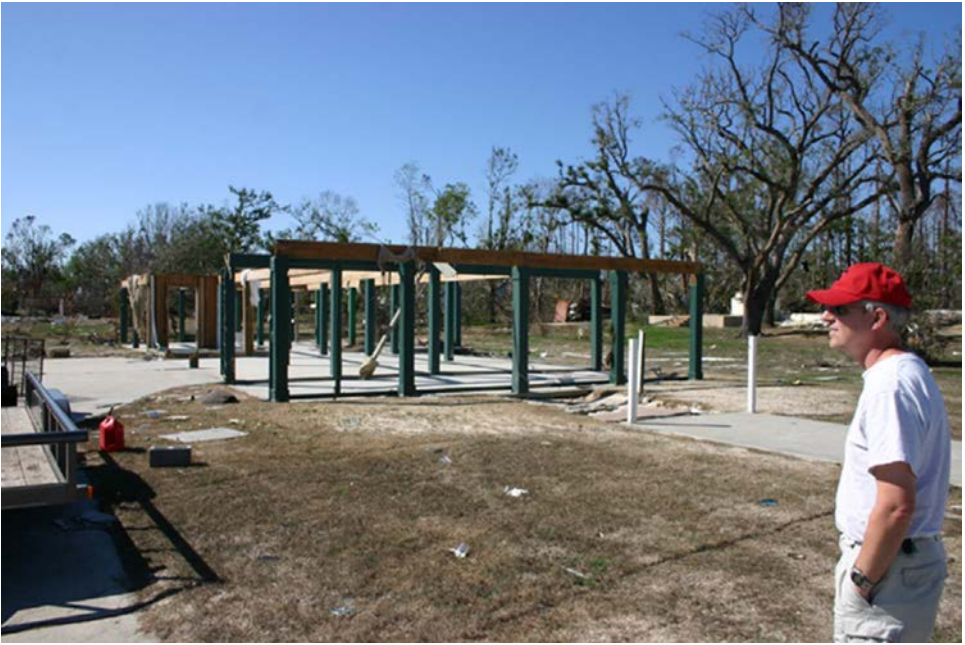
Remains of Rear Admiral Dave Titley's house after a nine-meter storm surge on the Gulf of Mexico
