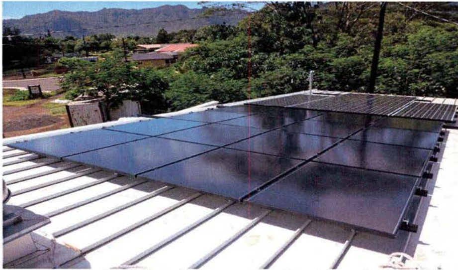
Figure 3. Kawaikini East classroom, East Kauai, showing two PV systems both connected in string configuration, CIGS (top) and monocrystalline (bottom).
