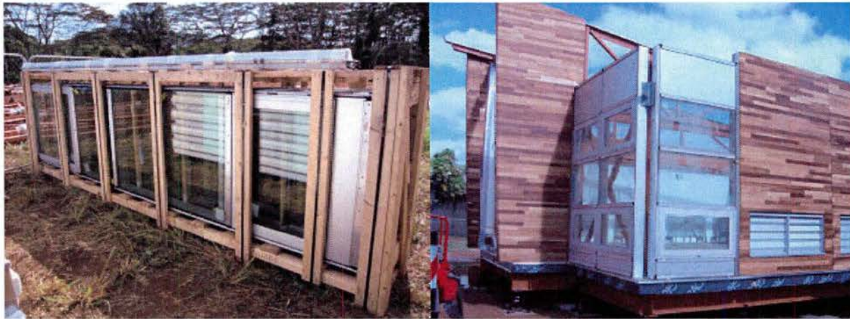
Figure 4.5.8 Crated curtain wall components at Ilima (l) and installed curtain wall at Kawaikini (r)
