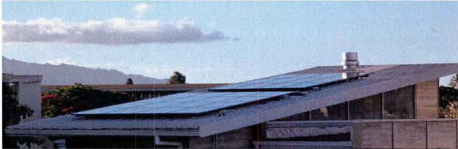
Figure 1. Ilima classroom, South Oahu showing the two PV systems installed to compare heterojunction with intrinsic thin layer (HIT) to thin film made of copper, indium, Gallium and diselenide (CIGS), both in a string configuration. HIT is located on top and CIGS at the bottom.
