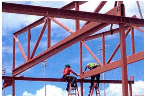
Figure 4.5.5 Installation of steel frame
