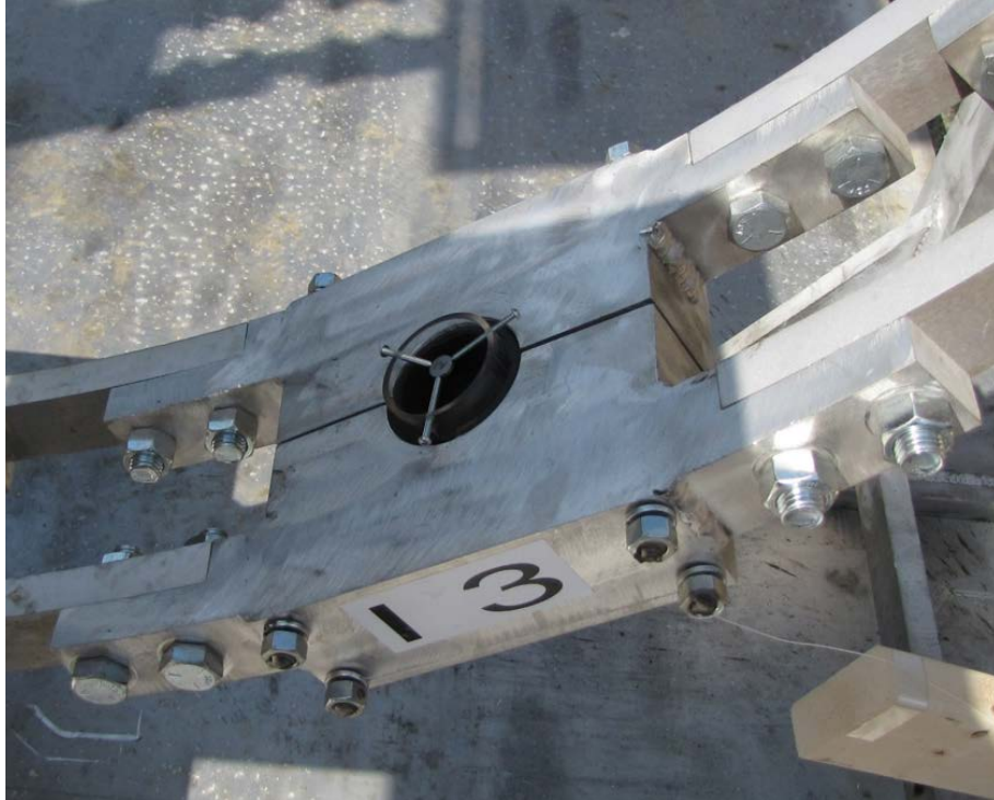
Fig. 3 Mounting of the blast gauge inside the Interior (I)-3 source location of the MEFCT support structure
