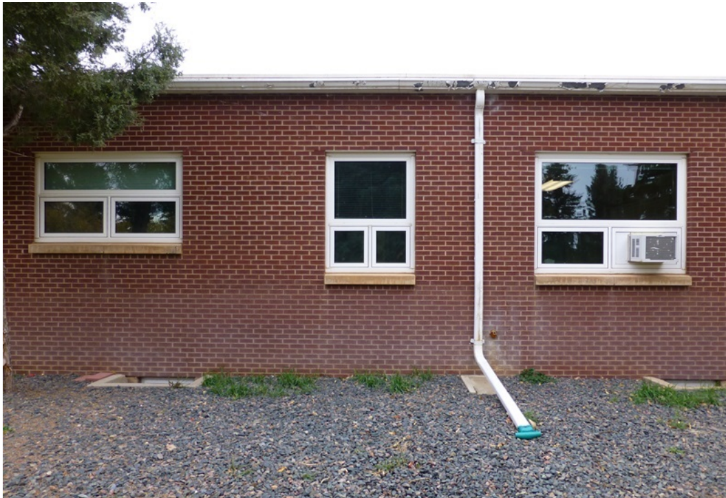
Photo 5. Laramie Armory, three window openings with replacement windows on the left side of the (front) elevation (ERDC-CERL, 2015).
