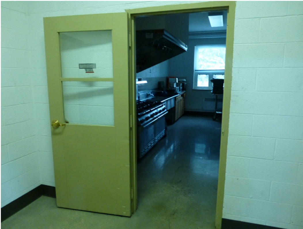
Photo 45. Laramie Armory, original metal door with glass panes, leading into the kitchen (ERDC-CERL, 2015).
