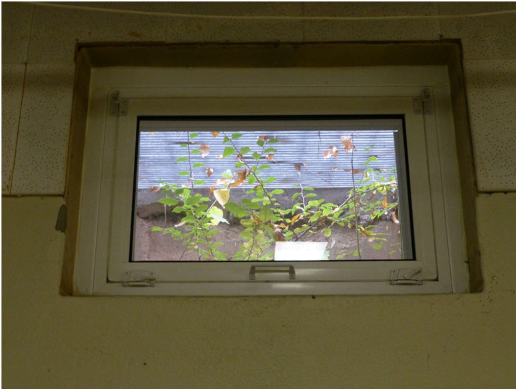
Photo 83. Laramie Armory, replacement vinyl hopper window in the basement (ERDC-CERL, 2015).
