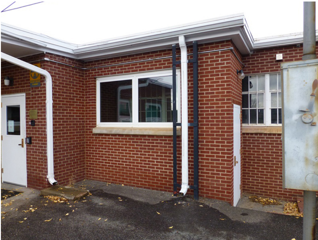
Photo 19. Laramie Armory, close-up of modified brick-enclosed basement entry on the east elevation (ERDC-CERL, 2015).
