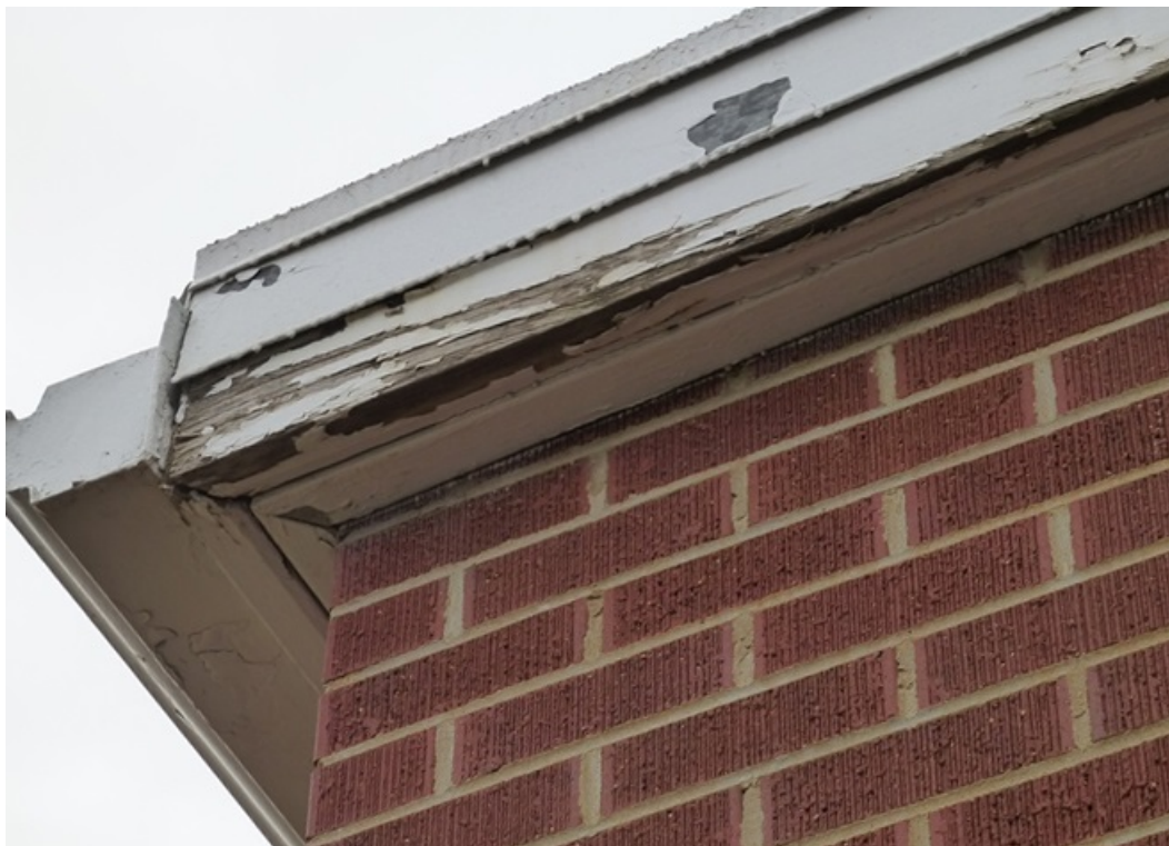
Photo 12. Laramie Armory, close-up of the wood/metal fascia and soffit system on the west elevation (ERDC-CERL, 2015).
