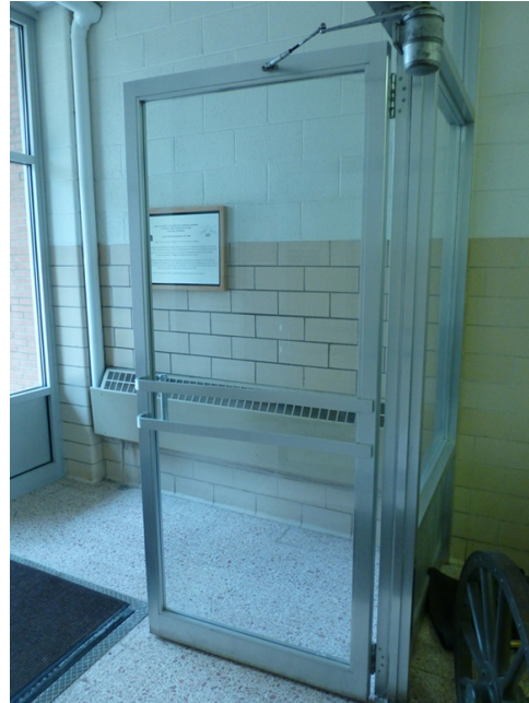
Bright-aluminum and plate-glass vestibule doors with sidelights and transom.
