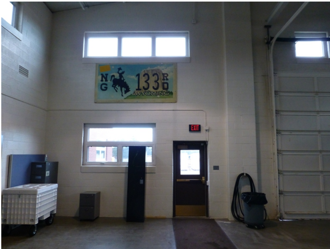
Photo 51. Laramie Armory, replacement door, window, and clerestory window on the left side of the west wall of the drill hall (ERDC-CERL, 2015).
