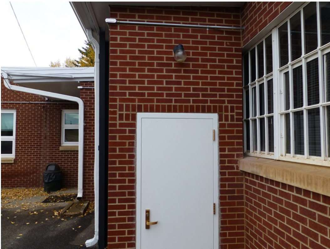
Photo 18. Laramie Armory, close-up of the modified brick-enclosed basement entry on the east elevation (ERDC-CERL, 2015).
