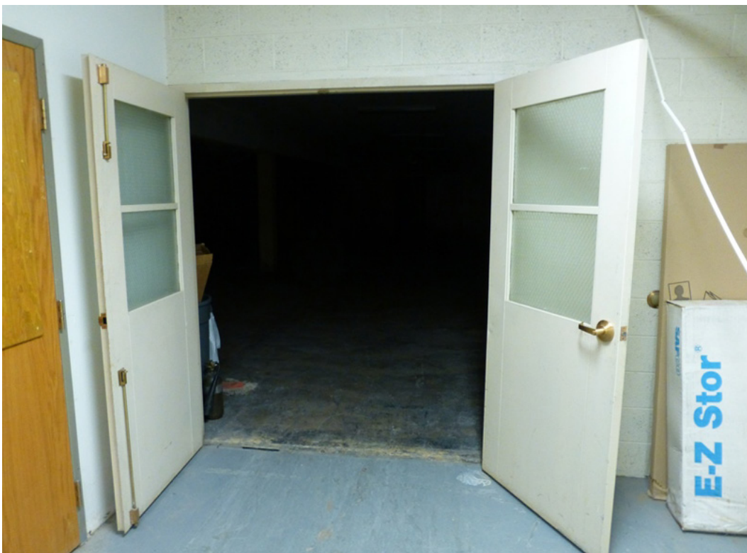
Photo 80. Laramie Armory, original metal doors with glass panes, in the basement (ERDC-CERL, 2015).
