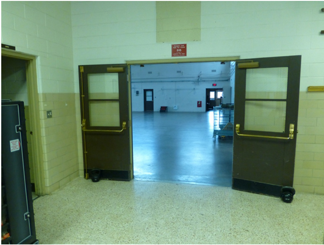
Photo 35. Laramie Armory, original metal doors with glass panes, leading from the lobby into the drill hall (ERDC-CERL, 2015).
