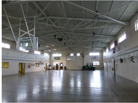
Open double-height drill hall space with concrete floors, concrete block walls, and exposed steel structure.
