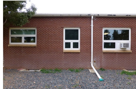
Three different size multipane steel-sash windows: original drawing from 1957 [left], compared to the condition of the different sizes vinyl one-over-two replacement windows in 2015 [right] (ERDC-CERL, 2015).
