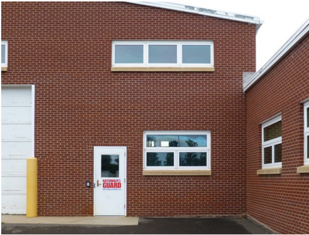
Photo 11. Laramie Armory, close-up of replacement window, clerestory window, and door on the west elevation (ERDC-CERL, 2015).
