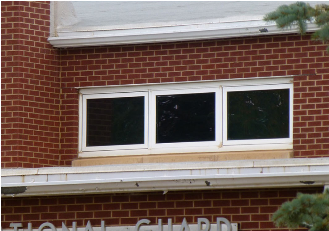
Photo 9. Laramie Armory, close-up of the replacement clerestory windows on the right side of the south (front) elevation (ERDC-CERL, 2015).
