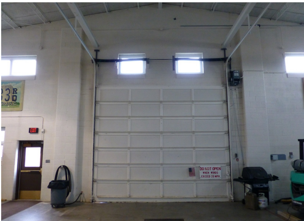
Photo 52. Laramie Armory, replacement metal overhead door on the west wall of the drill hall (ERDC-CERL, 2015).
