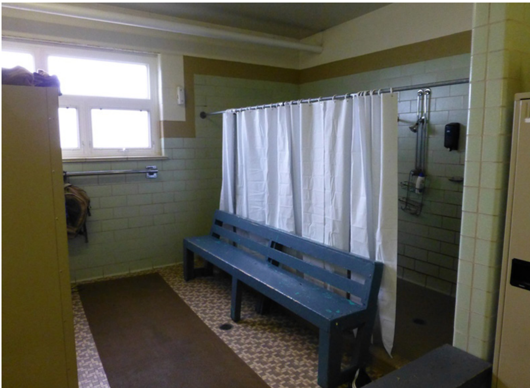
Photo 68. Laramie Armory, men's latrine with original shower stalls and glazed sanitary tile (ERDC-CERL, 2015).
