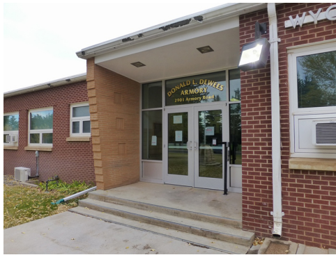
Recessed main entry with bright aluminum and plate glass doors, with sidelights, a transom, and a decorative brick wall framing the entry.
