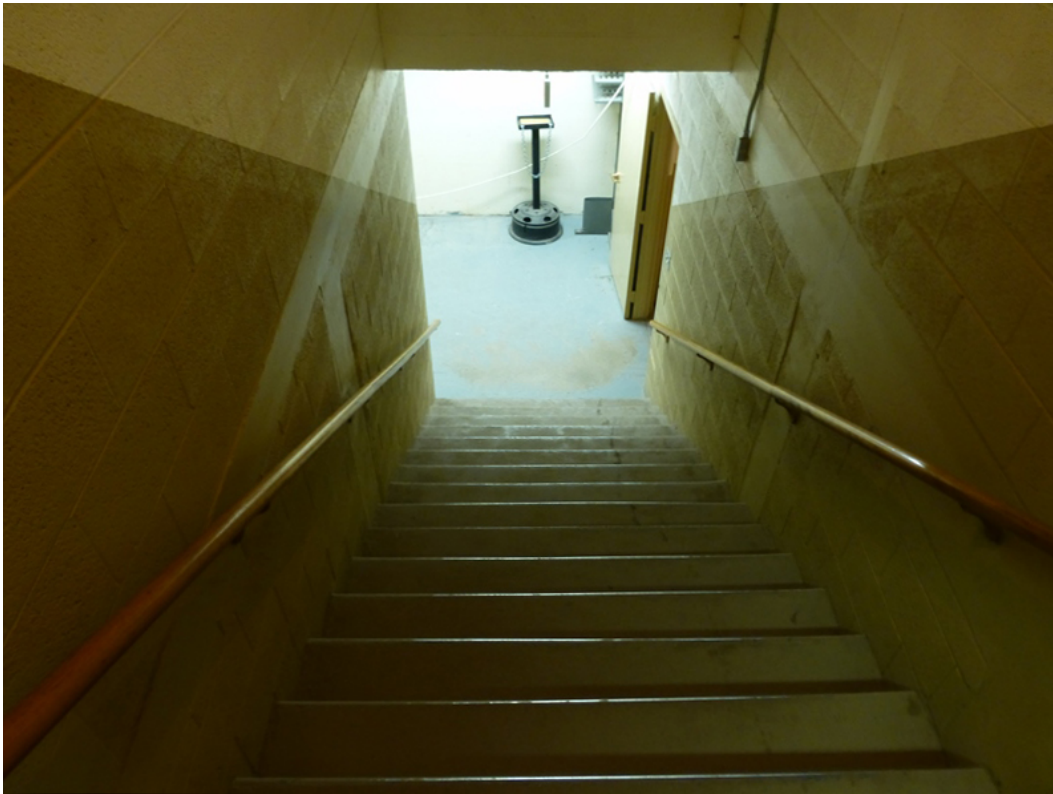
Photo 79. Laramie Armory, concrete staircase with original wood handrails, leading to the basement (ERDC-CERL, 2015).
