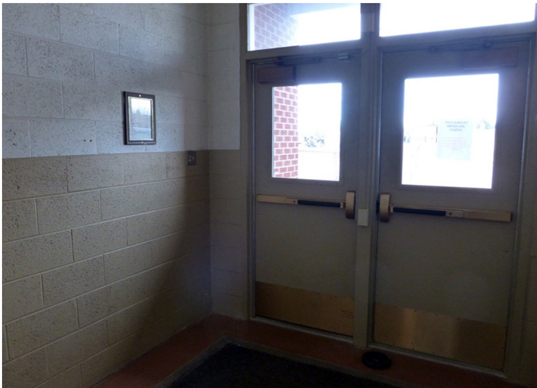
Photo 72. Laramie Armory, replacement metal doors, leading from north vestibule to the exterior (ERDC-CERL, 2015).
