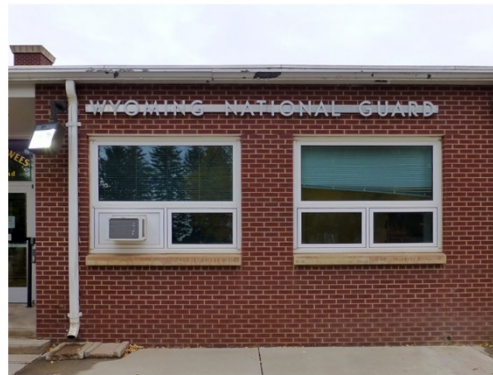
Eight-pane steel-sash windows and stainless-steel lettering on the south (front) elevation: Original drawing from 1957 [left], compared to the condition of the replacement vinyl one-over-two windows and original lettering in 2015 [right] (ERDC-CERL, 2015).
