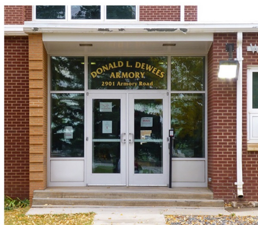
Main entry on the south (front) elevation: original drawing from 1957 [left], compared to the condition of the elevation with doors, sidelights, and transom in 2015 [right] (ERDC-CERL, 2015).
