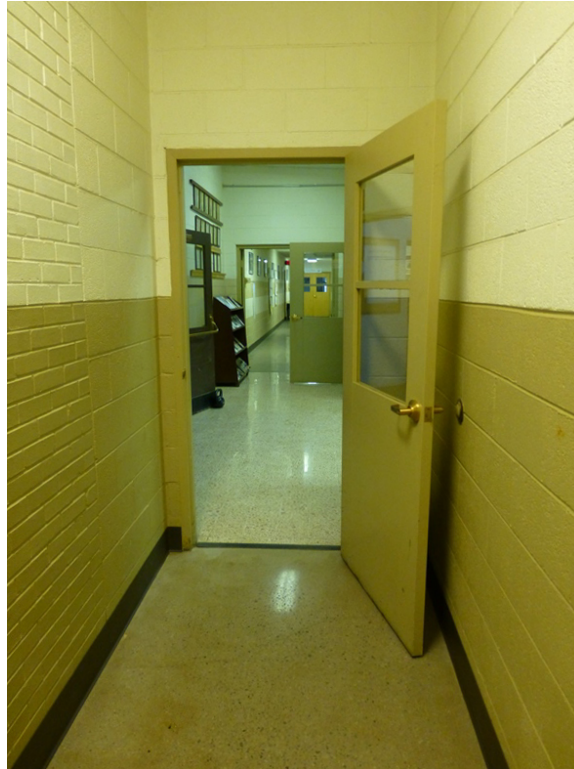
Photo 41. Laramie Armory, view from the west hallway toward the lobby, with exposed concrete floor in the foreground and original terrazzo floor in the background (ERDC-CERL, 2015).
