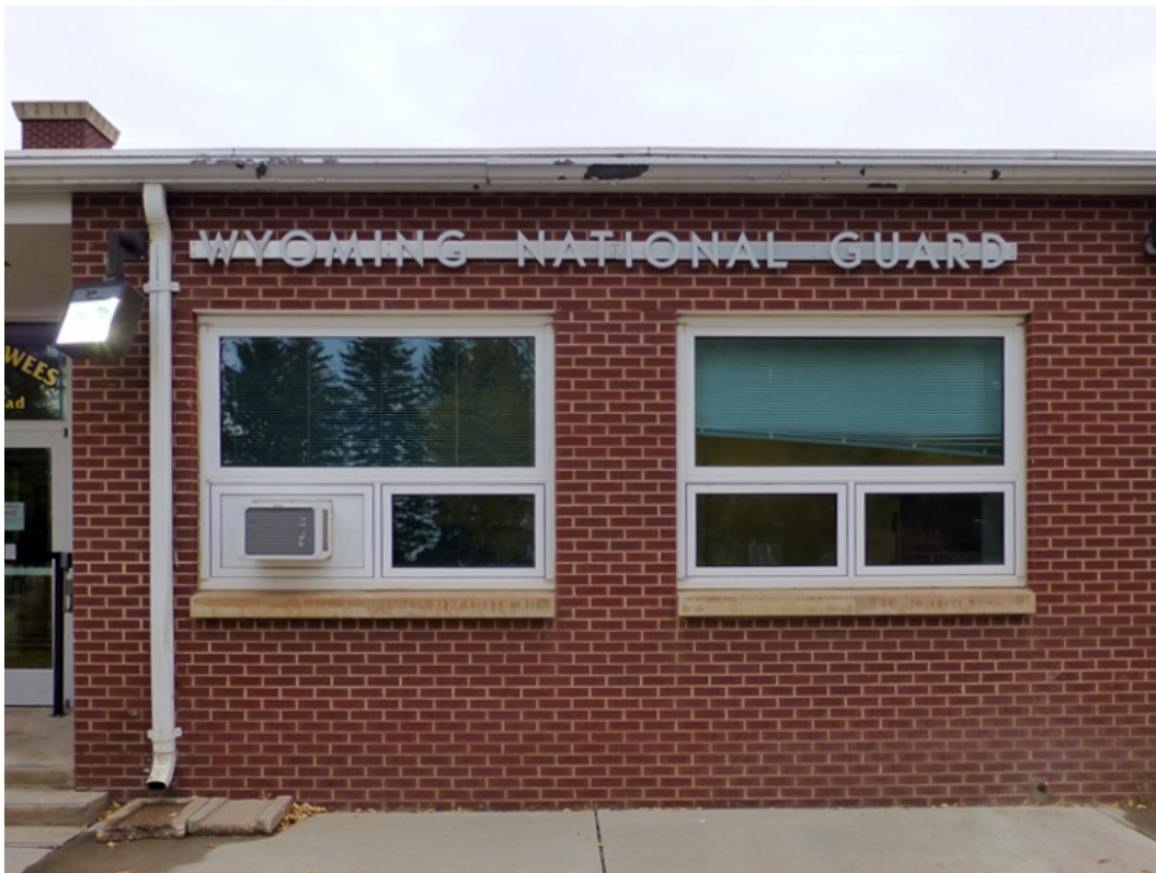
Photo 8. Laramie Armory, replacement windows, concrete windowsills, and stainless steel lettering to the right of the main entry on the south (front) elevation (ERDC-CERL, 2015).
