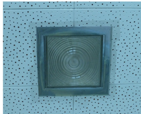
Square recessed light fixture: original drawing from 1957 [left], compared to the condition of the original light fixture located in the vestibule and lobby in 2015 [right] (ERDC-CERL, 2015).
