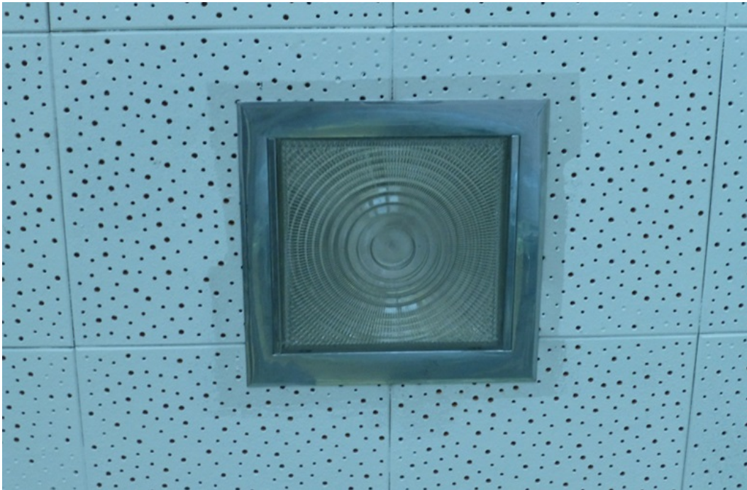
Photo 23. Laramie Armory, close-up of original acoustic tile ceiling and square ceiling light fixture in the south vestibule (ERDC-CERL, 2015).
