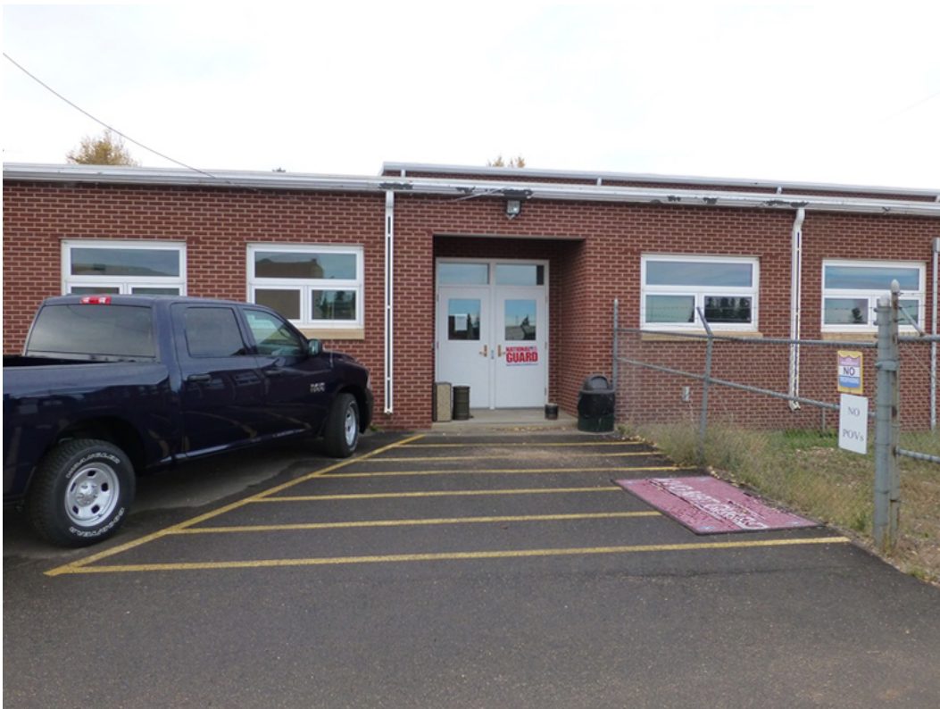
Photo 14. Laramie Armory entry, with replacement doors and transoms and replacement windows on the north (rear) elevation (ERDC-CERL, 2015).
