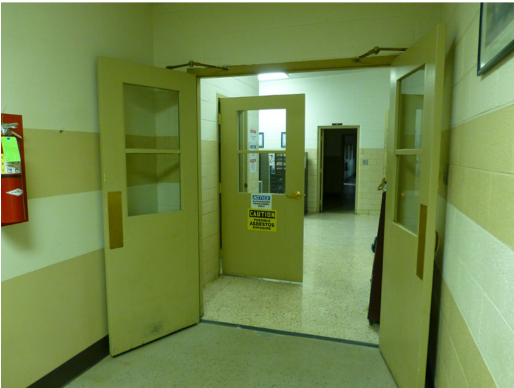
Photo 34. Laramie Armory, original metal doors with glass panes, leading from the east hallway into the lobby space (original metal door in background leads to the basement) (ERDC-CERL, 2015).
