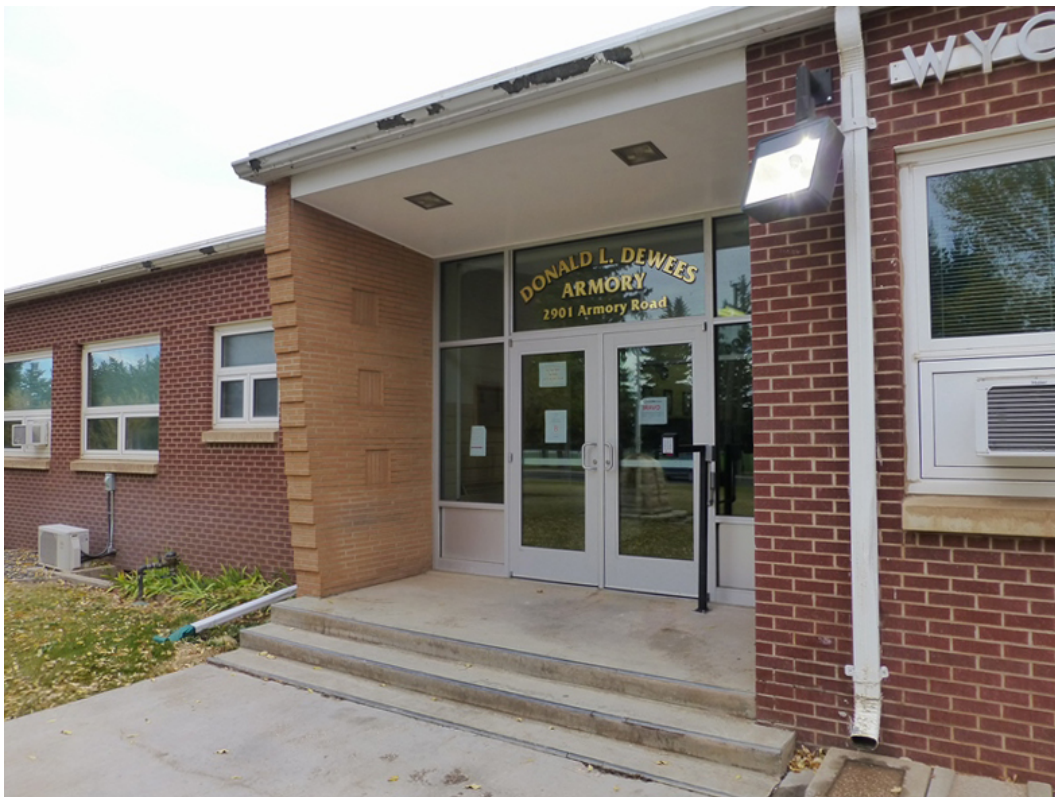
Photo 2. Laramie Armory, main entry with bright-aluminum and plate-glass doors with sidelights, transom, and a brick detail wall (ERDC-CERL, 2015).
