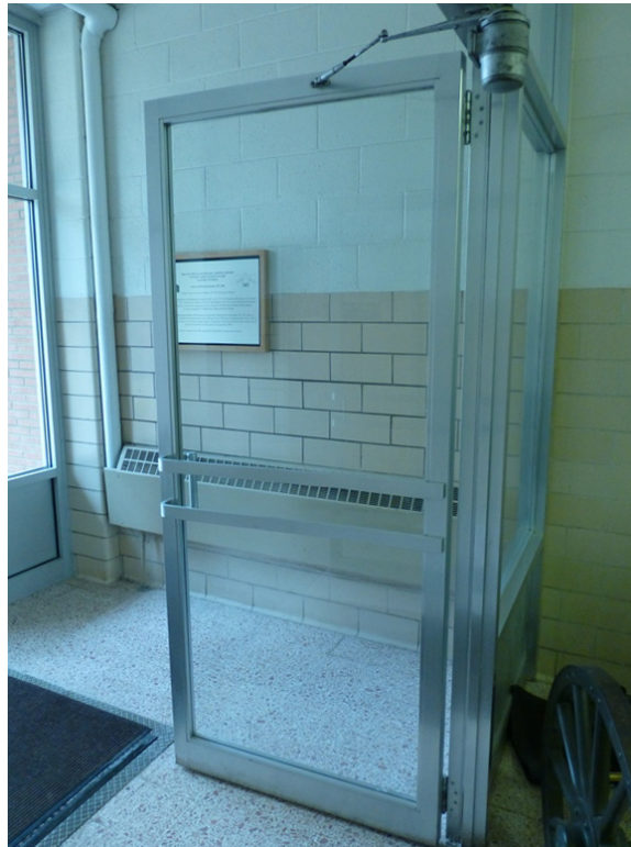
Photo 21. Laramie Armory, original bright-aluminum and plate-glass vestibule doors (ERDC-CERL, 2015).
