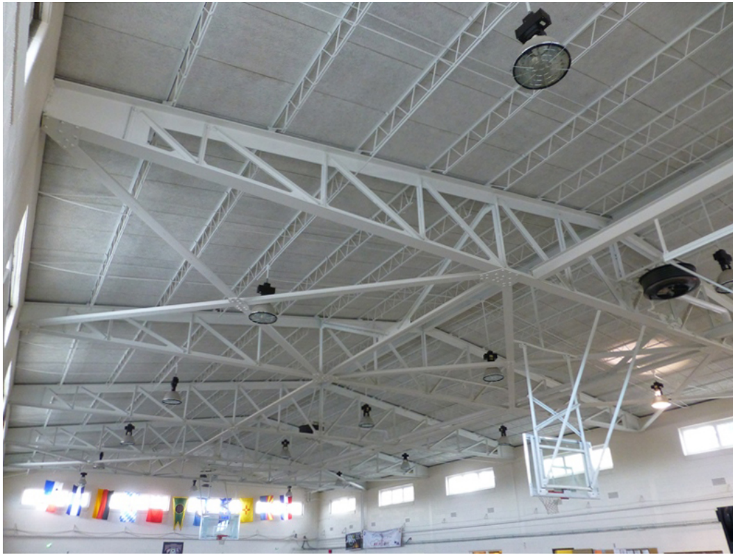
Photo 55. Laramie Armory, exposed metal truss roof system in the drill hall (ERDC-CERL, 2015).
