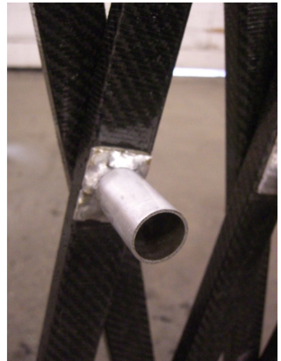
Figure 6: Incorporating a protruding nub into the joint design allows it to interface with the planking.
