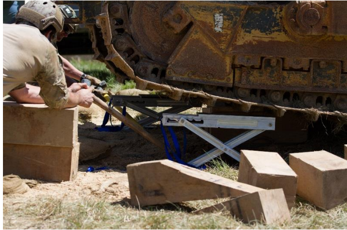
Figure 8: Autoshore Ninjas shoring D6 Bulldozer
