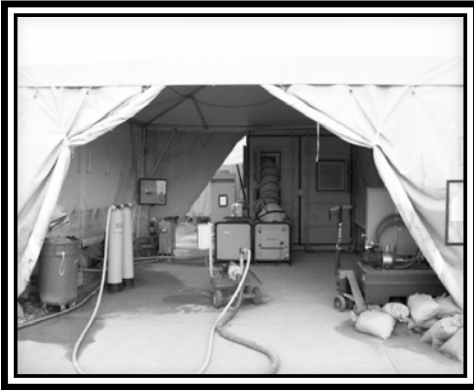
Potable Water Feed to EWPS
