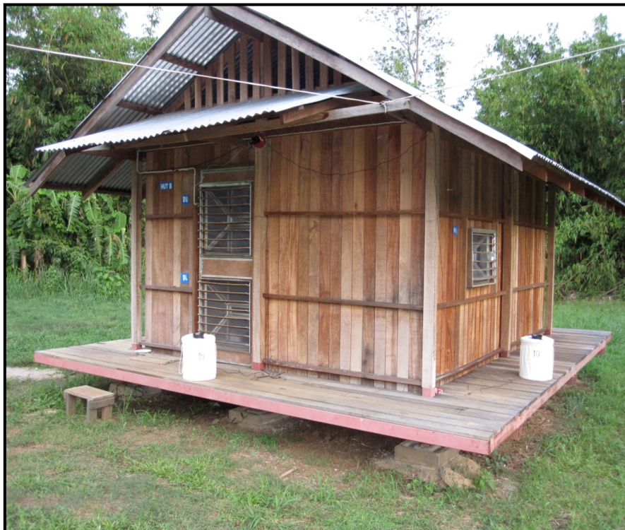
Figure 9. Experimental hut with 50 m 3 room volume. The interior hut dimension resembles a rectangle (4 m wide x 5 m deep x 2.5 m high). During sample collection doors and windows remained closed but all door and window louvers were fully opened.
