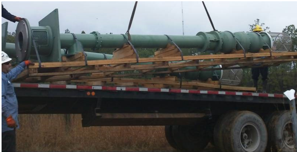
Figure 6. New pump components being installed at Fort Polk CVWF.
