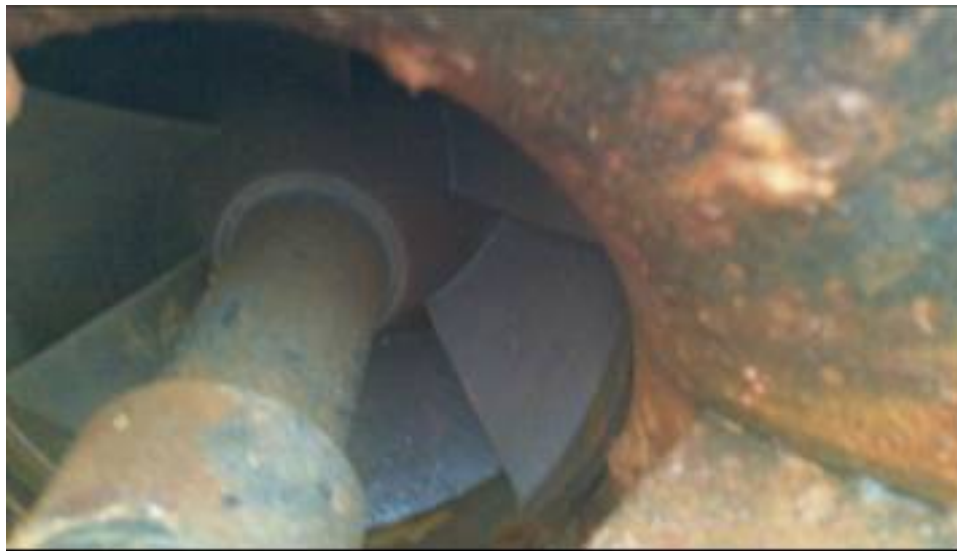
Figure 15. Old Unit 2 pump first-stage impeller.
