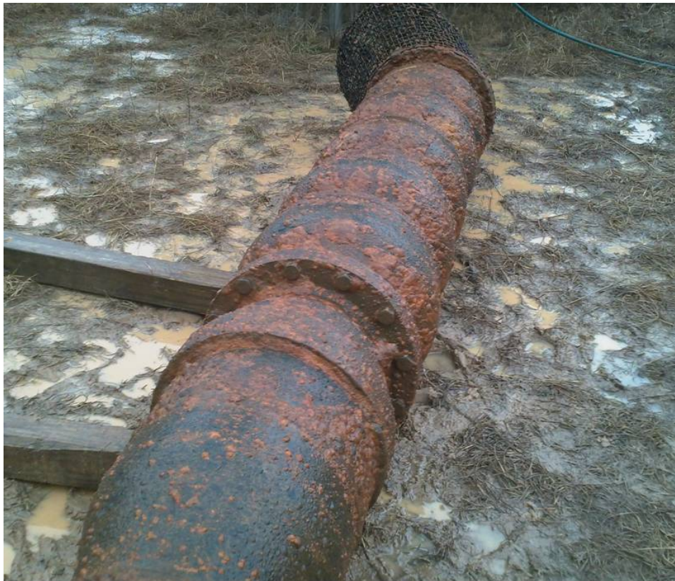
Figure 16. Condition of old Unit 1 pump bowls.
