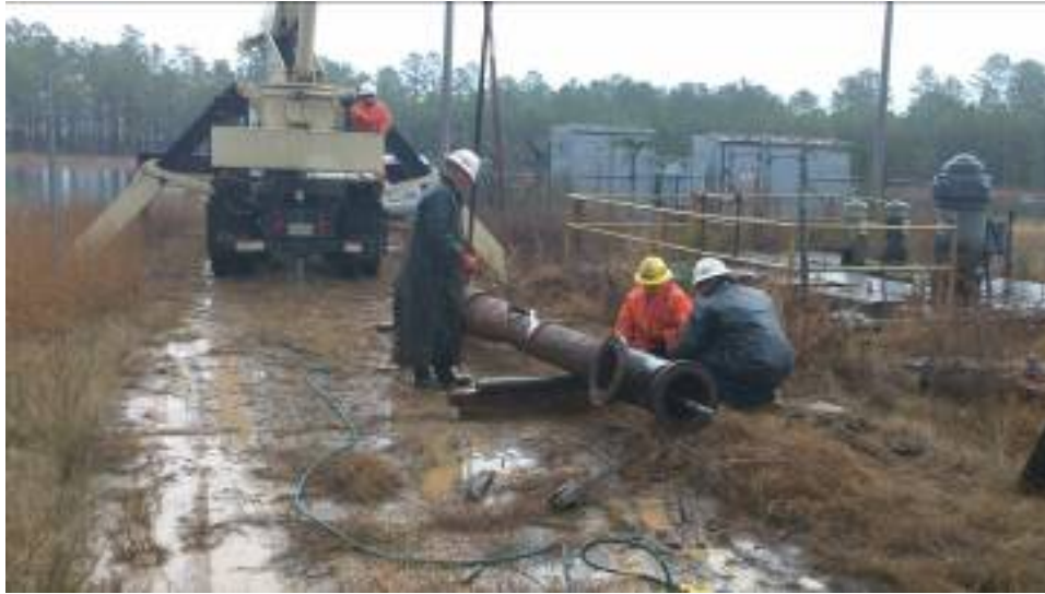
Figure 7. Old (inoperable) Unit 2 pump disassembly.
