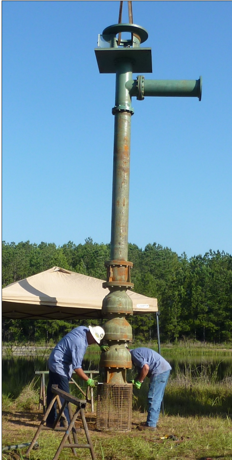
Figure 23. Condition of outer surfaces of Unit 1 pump, after 15 months of service.
