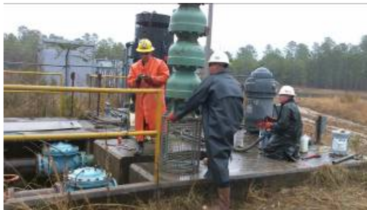
Figure 10. New Unit 1 pump strainer basket installation.
