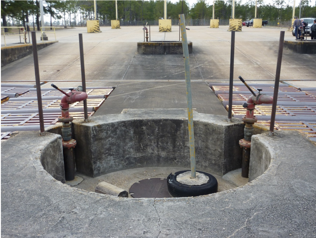
Figure 2. Water cannons on CWVF central island.
