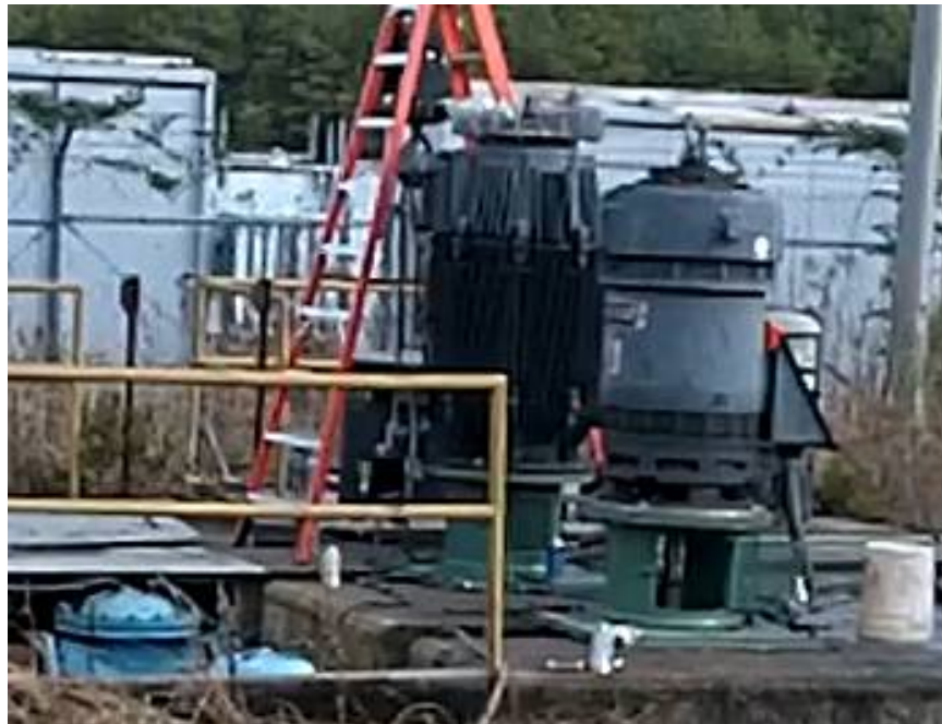
Figure 12. New Unit 1 pump installation with motor installed.
