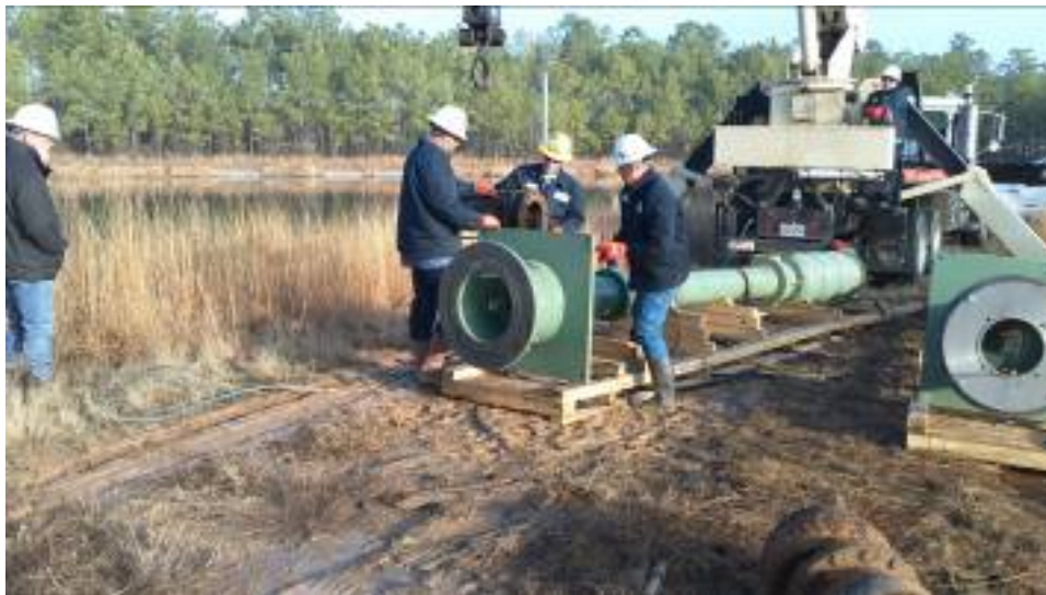
Figure 8. New Unit 2 pump header installation.
