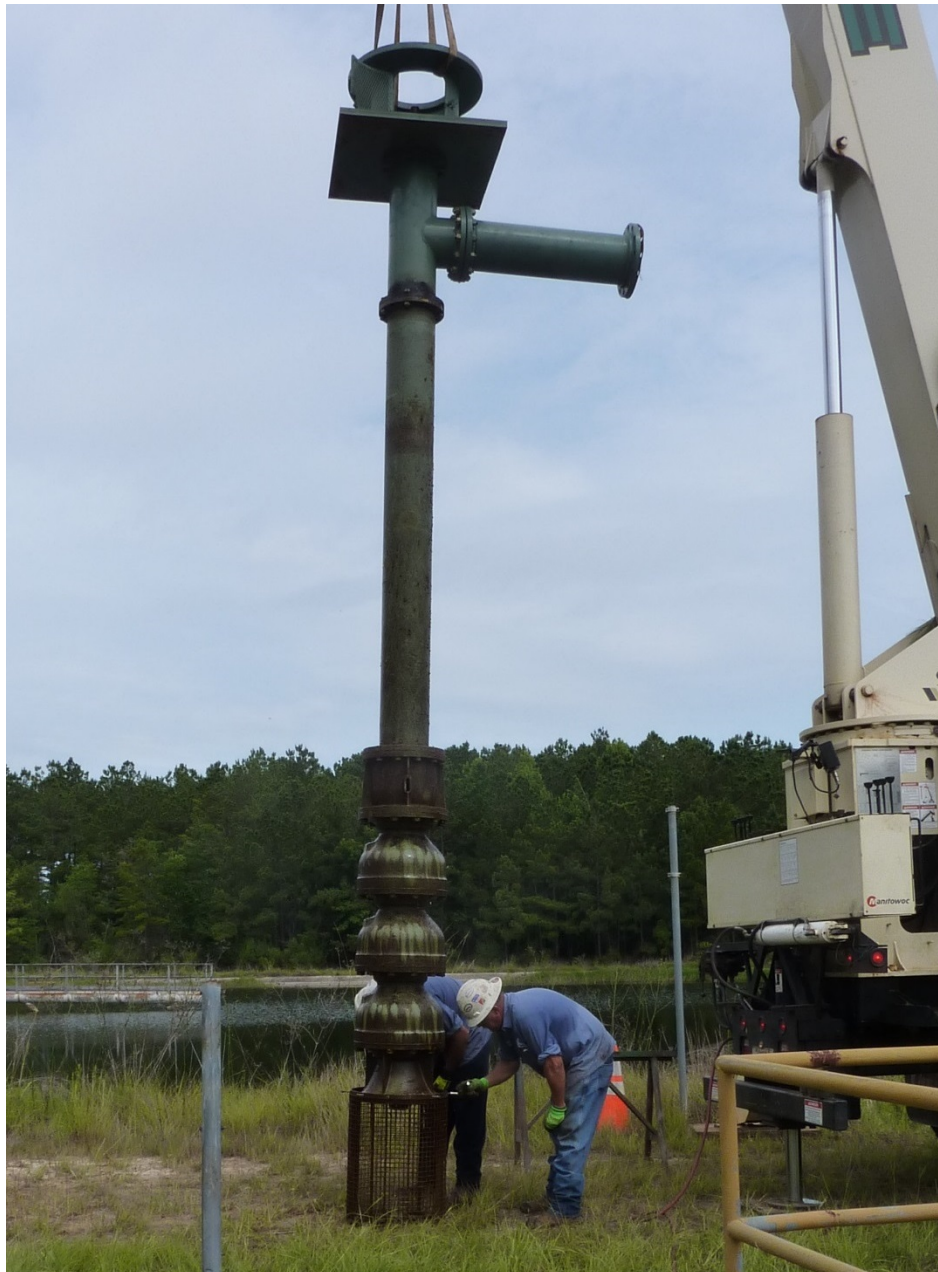
Figure 27. Condition of outer surfaces of Unit 2 pump after 15 months of service.
