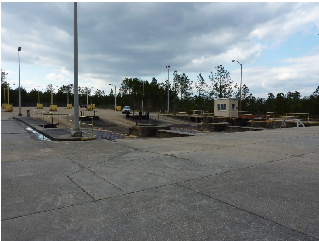
Figure 1. Prewash area at North Fort Polk CVWF.
