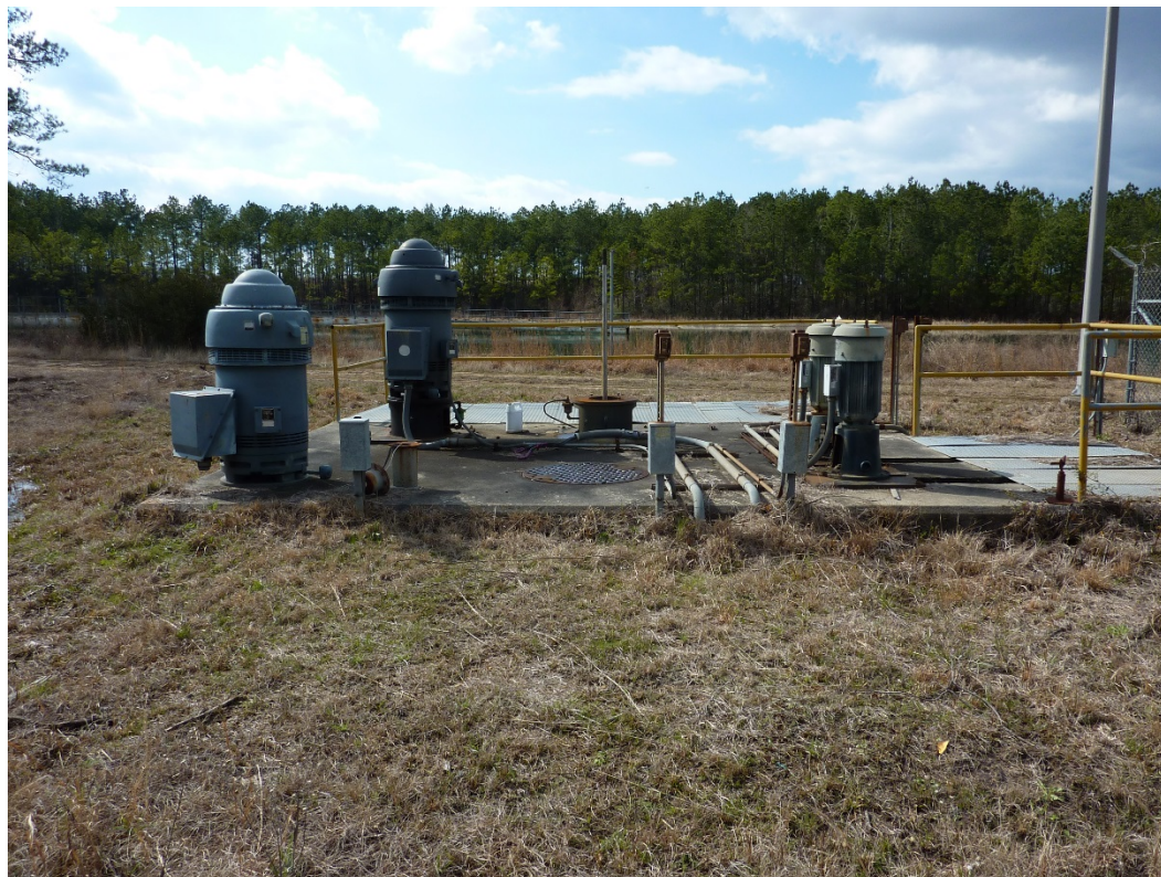
Figure 4. CVWF pumping station.
