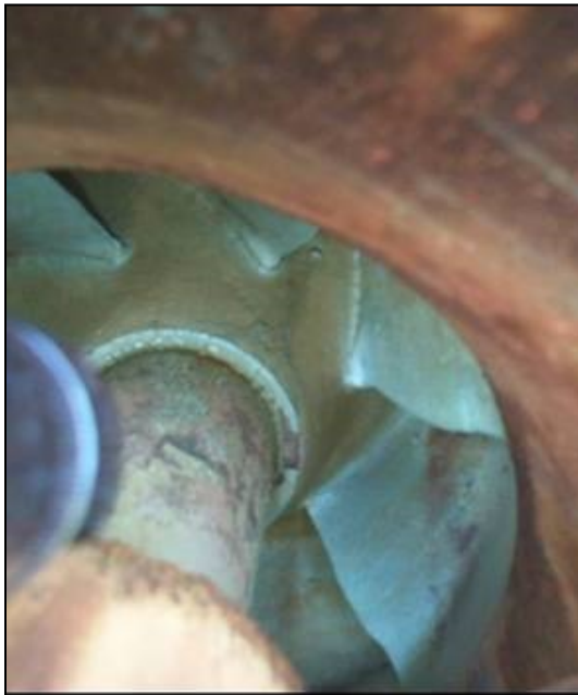
Figure 24. Condition of Unit 1 first-stage impeller, after 15 months of exposure.
