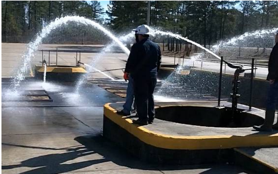
Figure 13. North wash rack in operation.
