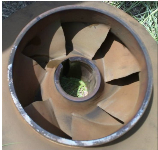
Figure 25. Condition of Unit 1 first-stage impeller after 15 months of exposure.
