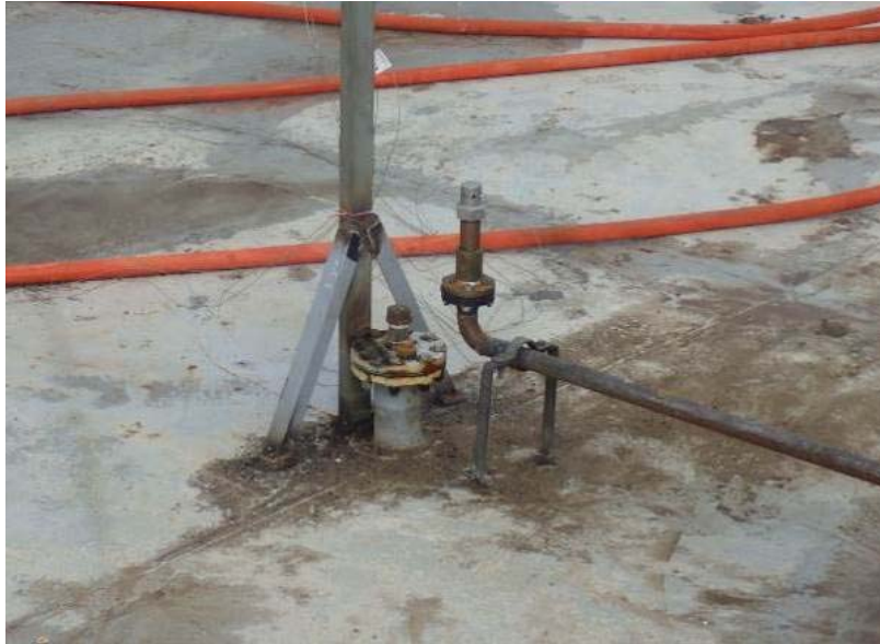
Figure 7. View of fuel nozzle.
