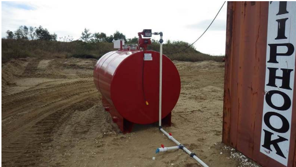
Figure 6. Fuel supply tank.
