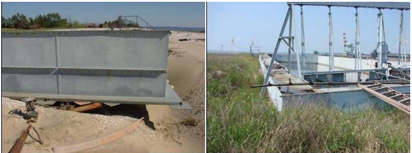
Figure 3. Burn pan showing sand removed from base and disconnected pipes (left) and other damage (right).
