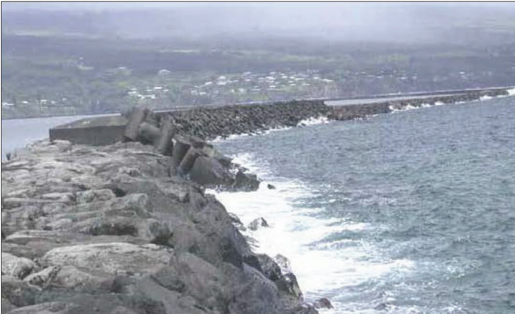
Figure 1-3. The breakwater with rib cap and tribar (view from east to west).
