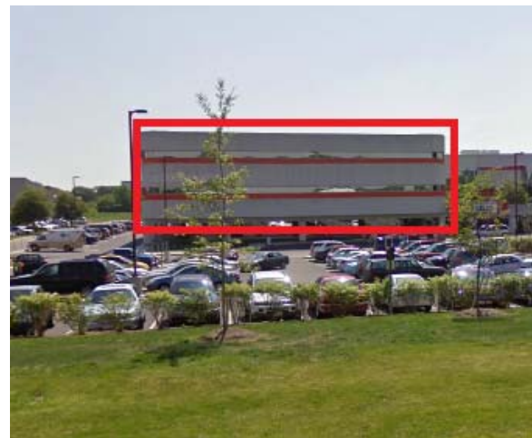
(b) Building I (parking garage)
