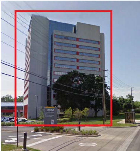
(c) Building II (office building)
