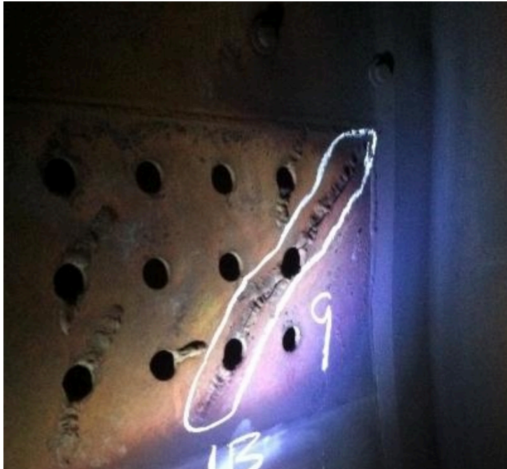
Figure 25. Exhaust Collector Vent Hole Cracks
