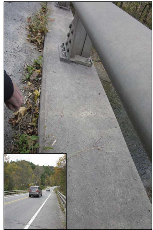
West Lebanon, NH, bridge curb repair, completed in December 2002, using antifreeze concrete
