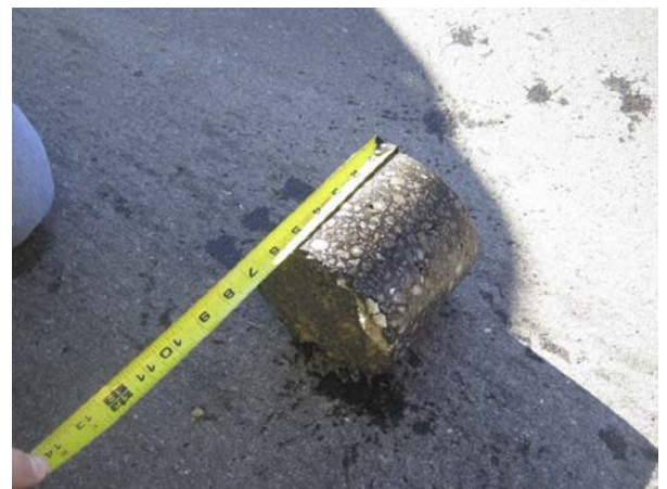
Cored asphalt concrete
