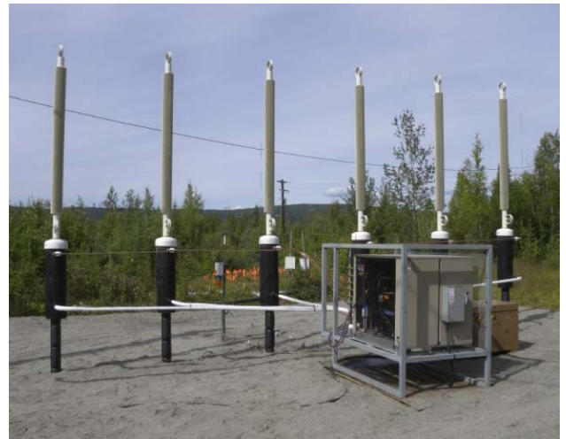
Hybrid thermosyphons installed in Fairbanks, AK
