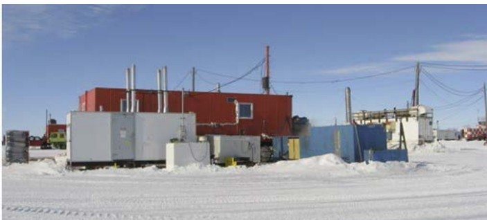
Incinerator and wastewater set up at Pegasus Runway, 2011–12.
