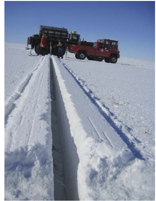
View of the trench used for installing temperature sensors in the runway
