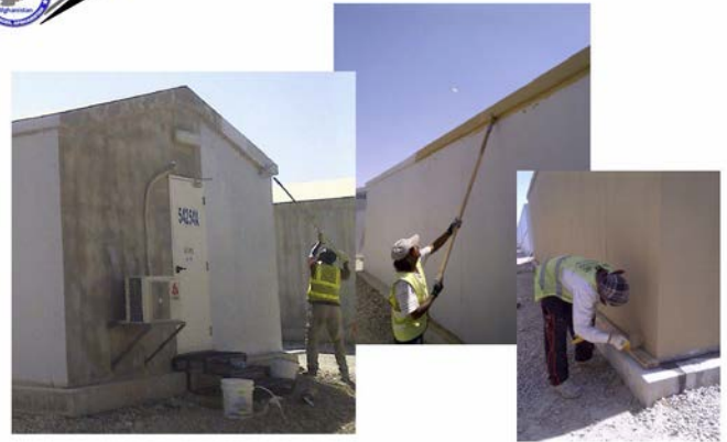
Exterior Sealant and Ceramic Paint
