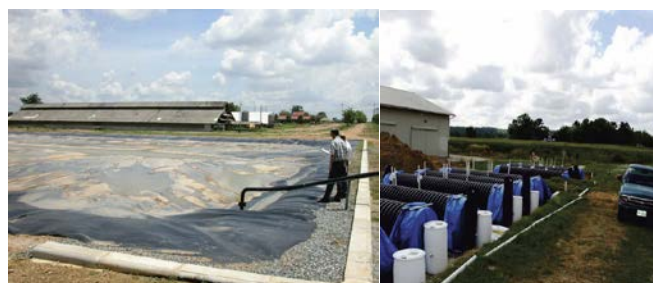
Examples of two simple anaerobic digester reactors: covered lagoon (left) and bag reactors (right)
