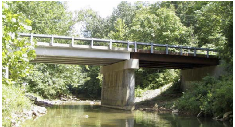
Fort Knox, KY Bridge 04 in 2013
