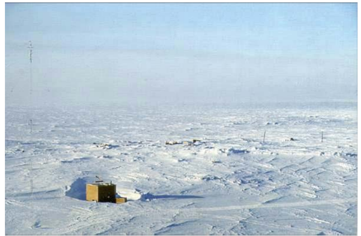
Amundsen-Scott South Pole Station entrance in 1970, completely buried by accumulated and drifted snow
