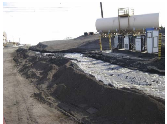
Drainage channel along the "Gasoline Alley" adjacent to the fueling station
