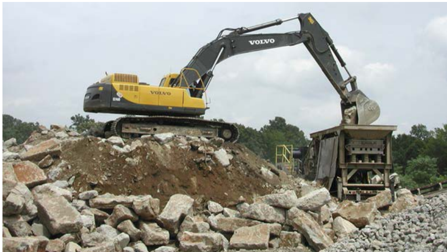
Concrete recycling with on-site crusher.
