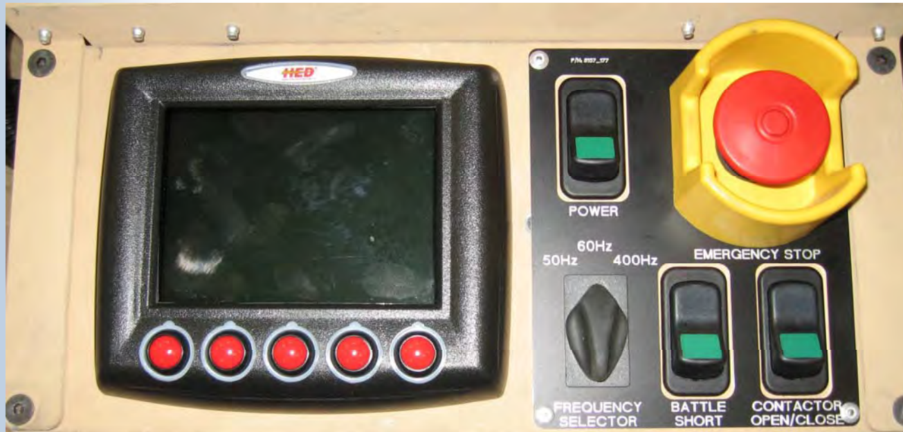
Operator Interface Panel
