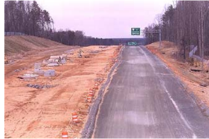
Poor lane markings
