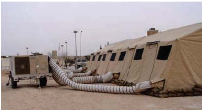
Marines use 3-in-1 unit to power, cool and heat field facilities, enabled by DAC
