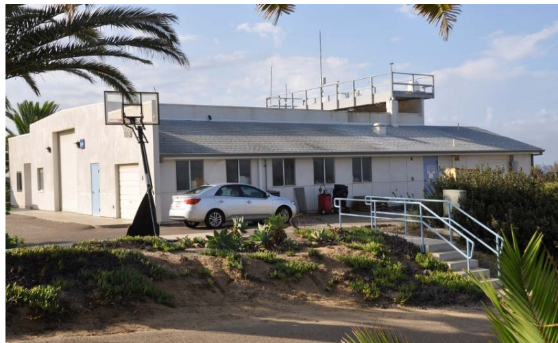
Figure 58. Commander Everett added the north wing machine shop lean-to addition (behind car) to Building F-36 in 1991, which was later expanded westward (to right of windows) as part of the contracted south-wing addition to the building (extreme left) in 2010.
