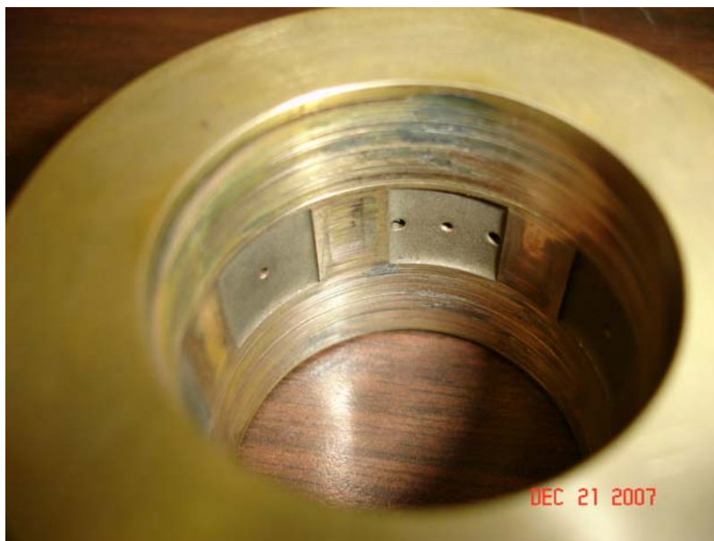
Fig. 27. Localized pitting and burnishing where loading was applied during testing.
