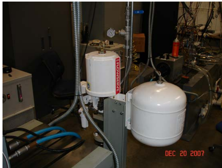
Fig. 14. Installed control valve.
