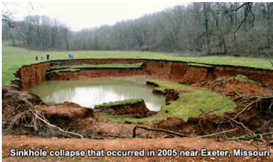
Figure 20. Sample sinkhole. (Source: http://blogs.mo.gov/geology/tag/sinkhole/ )
