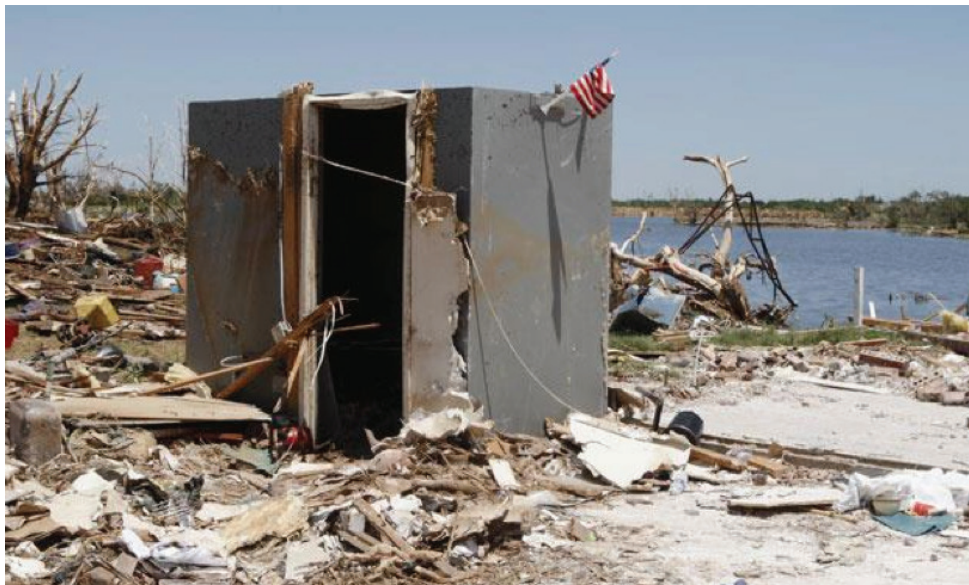
Figure 12. Safe room condition after a tornado hit Piedmont, Oklahoma. (Source: Syracuse Media Group webpage.)
