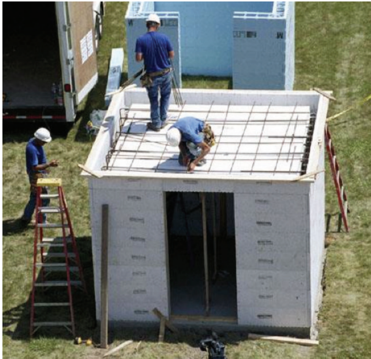
Figure 11. Safe room construction in Sioux City, Iowa. (Source: Dave Gatley, FEMA.)
