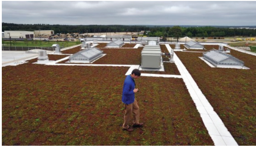
Figure 7. Green roof at the Transportation Deployment support area at Fort Bragg. (Source: LiveRoof Brand webpage.)
