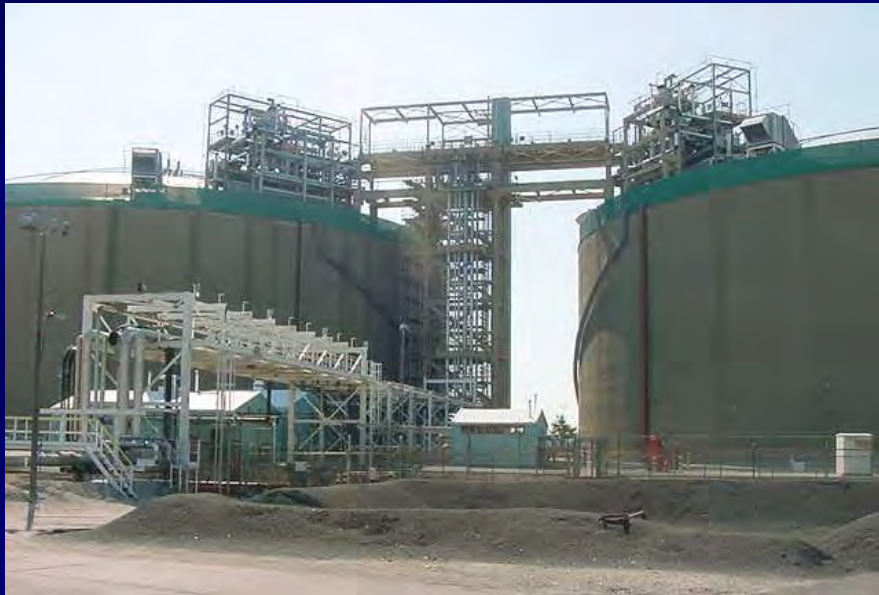
PGW PORT RICHMOND PLANT
