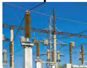
Utility Company Power
