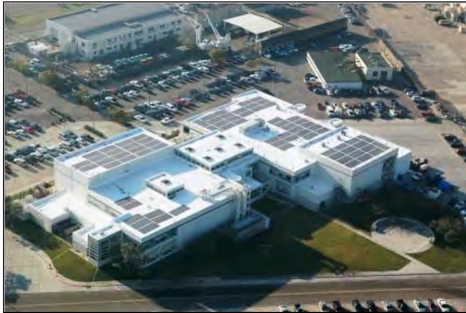
Naval Base Coronado - Building 352
