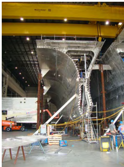
JHSV 2 and 3 Under Construction
