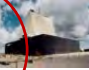
Early Warning Radar
