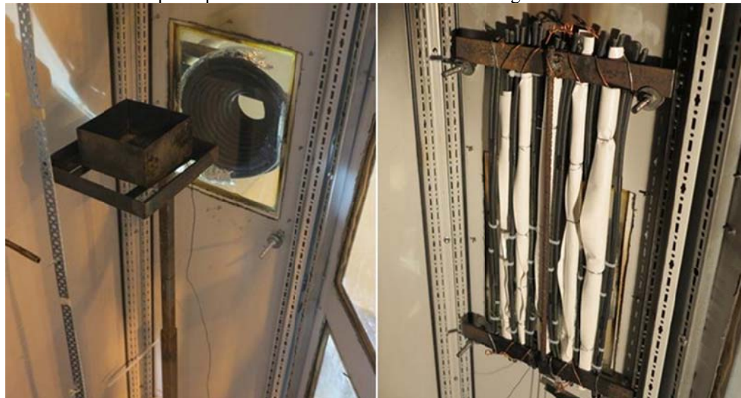
Figure 2. (Left) Position of heptane pool in fire scenario 1. An obstructing panel placed about 50 mm above the pan edge (see Figure 5). (Right) Cable ladder used in fire scenario 2.
