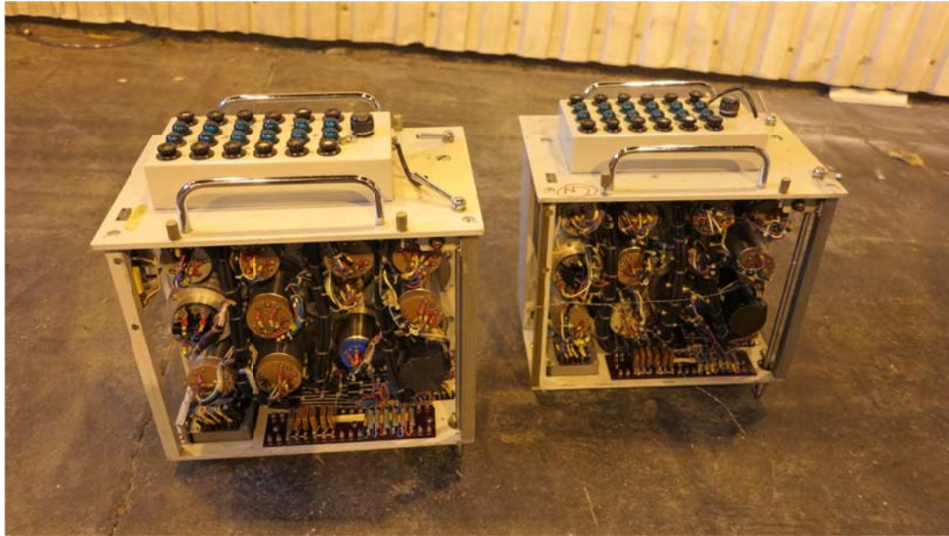
Figure 23 – Obstructions in the electrical cabinet
