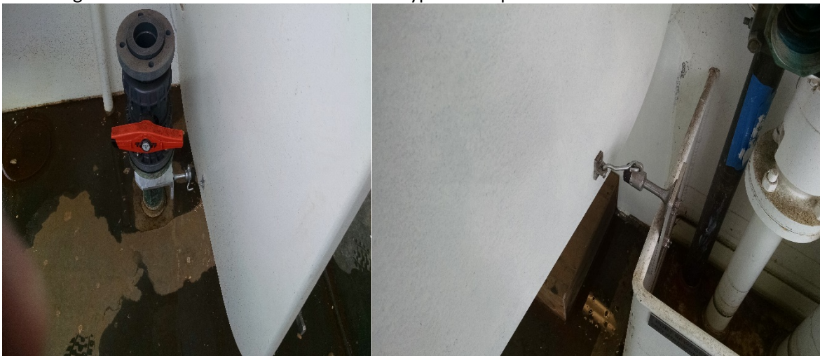
Door stops/holdbacks starting to be installed...these two on exterior doors don't seem correct. The hook is doing all the work. Not sure this is the best type of "stop" for this location. Will talk with Adam.
