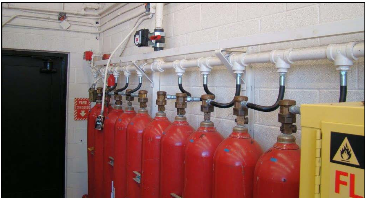
Figure 1. Automatic CO 2 fire suppression system.
