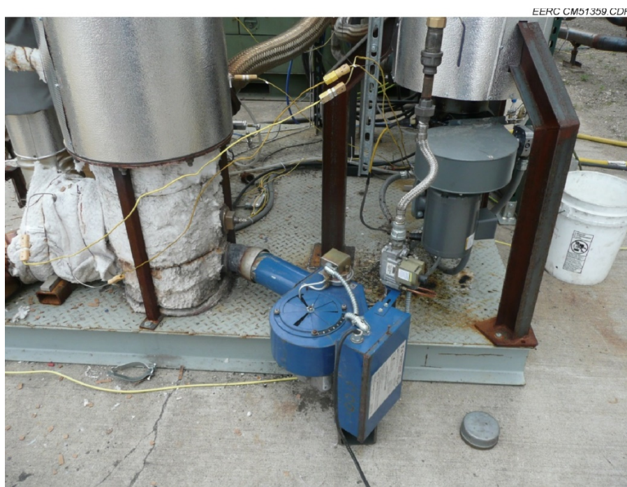
Figure 11. Natural gas-fired preheat combustor.
