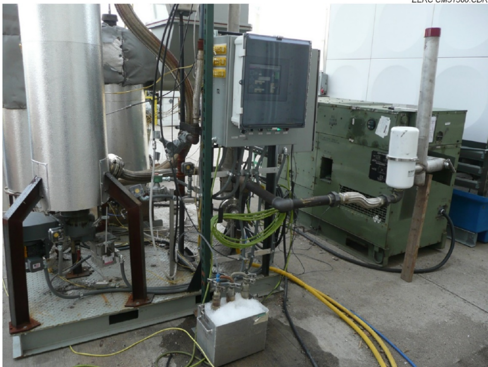
Figure 10. Photograph of the control panel and the syngas transfer line to the TQG.
