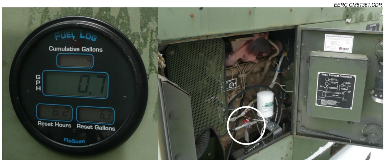
Figure 13. Sensing unit display of the fuel consumption meter, left, and one of two fuel flowmeters that were installed on the TQG, right.
