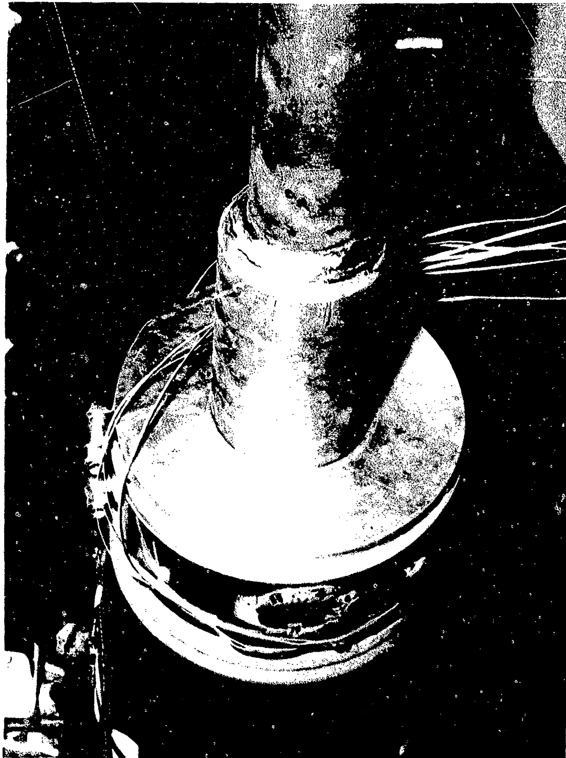
Figure 10. Installation of Strain Gages
