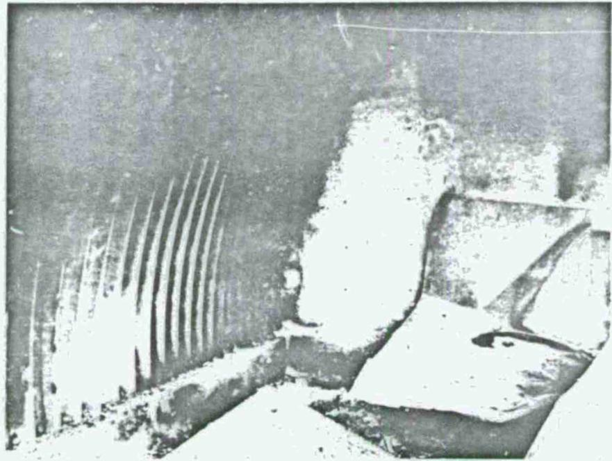
FIG. 38. Left Rear Corner of North Igloo. Scorching is evidence of burning of acceptor charges; circular pattern on wall is imprint of one end of an acceptor charge.
