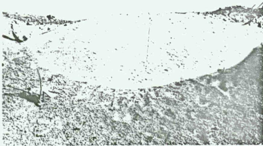
FIG. 42. Interior View of Concrete Rear Wall of East Igloo, Showing Acceptor Fragment Impacts.
