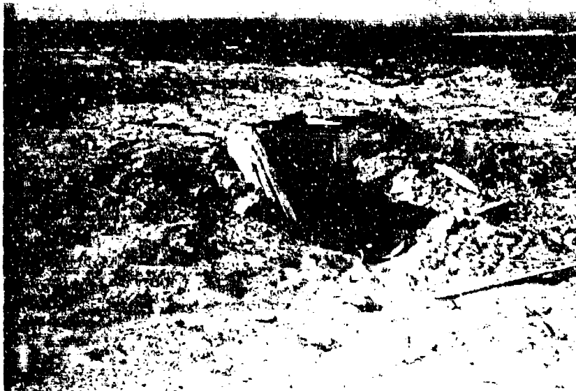
Fig. 4.1 Damage to Structure A-1 Due to Shot Baker (covered-trench below-grade)
