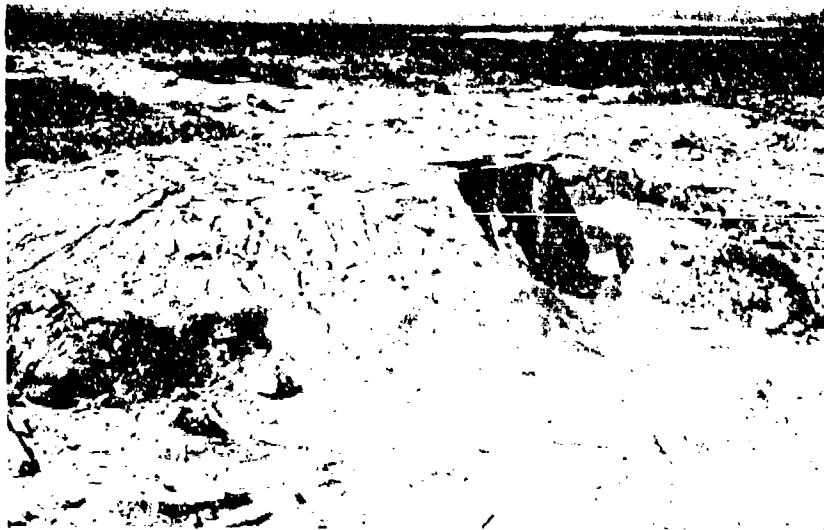
Fig. 4.2 Shelter A-2 After Shot Baker (covered- trench below-grade)
