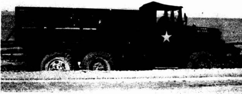
b. M35A2 (mod) was immobilized on 2d pass at Carson Sink site 2 (item 19)
