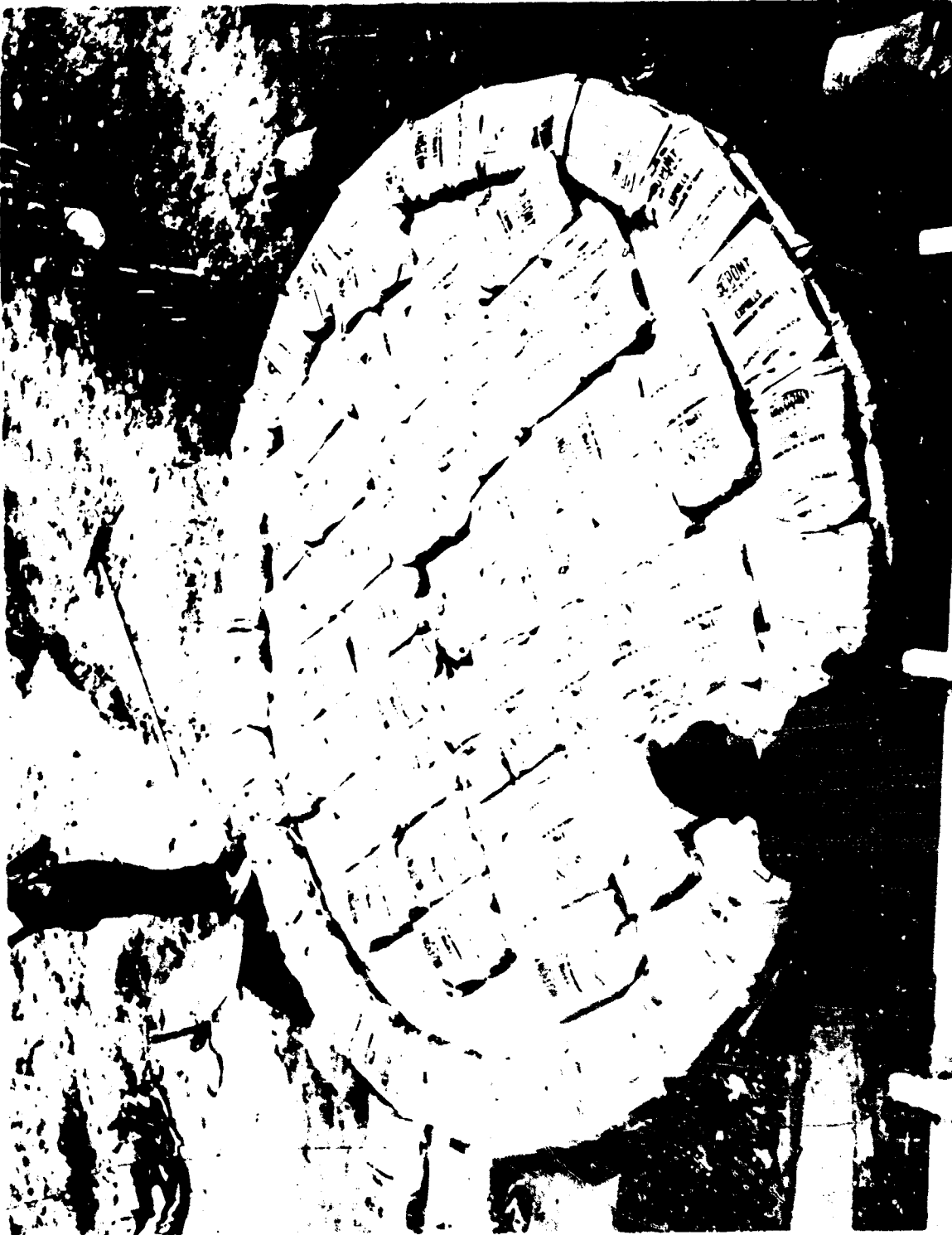
FIG. 24 EVENT 1, LAYER 2 PRIOR TO FILLING SPACES WITH LOOSE AN/FO
