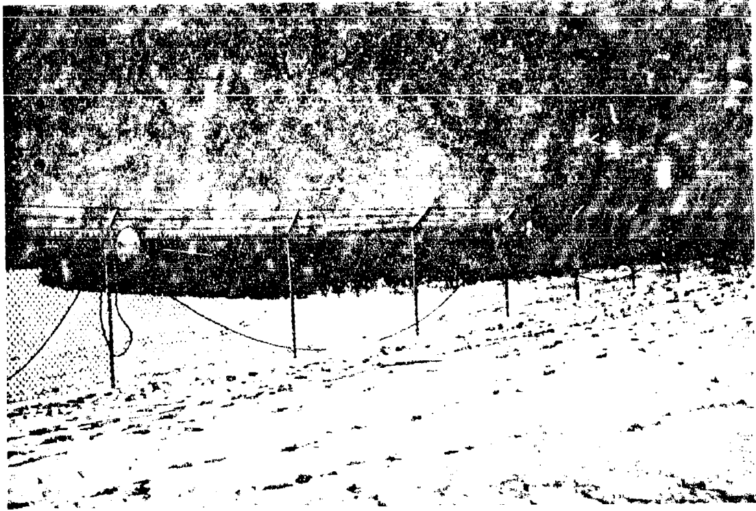
FIGURE NO. 1: Standard 100-Watt Light Fixtures, Approximately 6-Feet High and 10 Meters Apart
