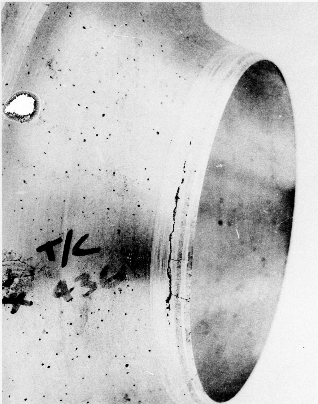
Figure 35. Close-up of Fracture in Cast Bellmouth Liner.
