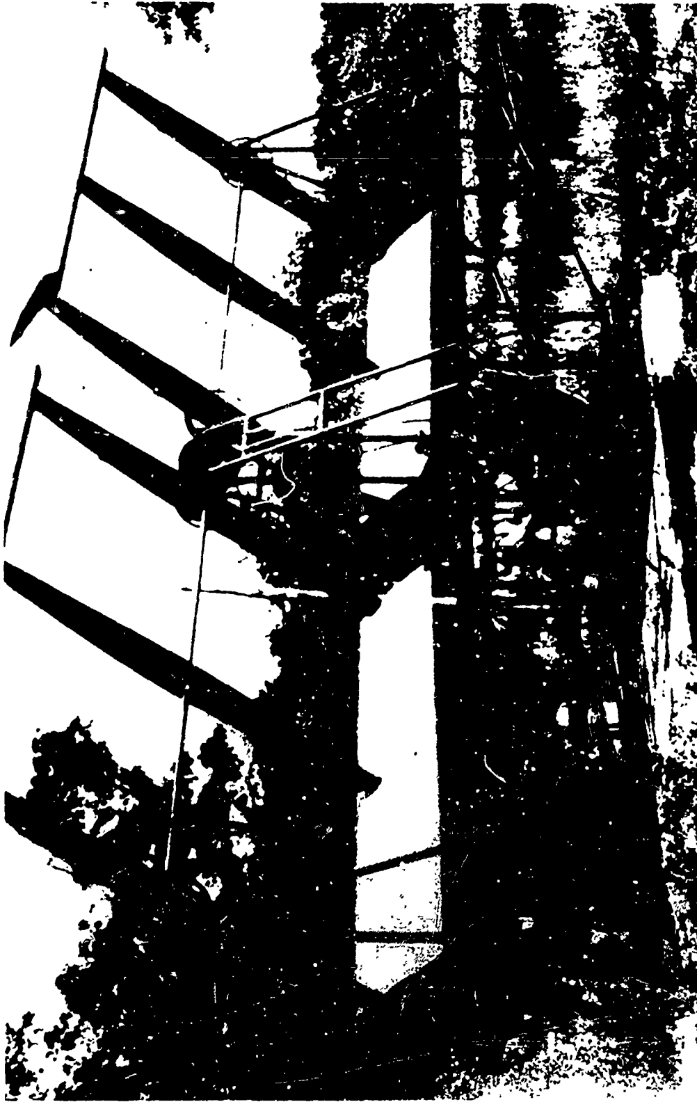
Figure 62. Unidentified (Nemeth, Ref. 12N) Full-Size Cyclogiro of the 1920's. Note Rotary Engine and Direct Chain Drive.
