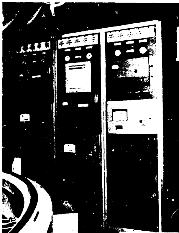
Figure 4. SYSTEM MONITORING AND CONTROL PANEL
