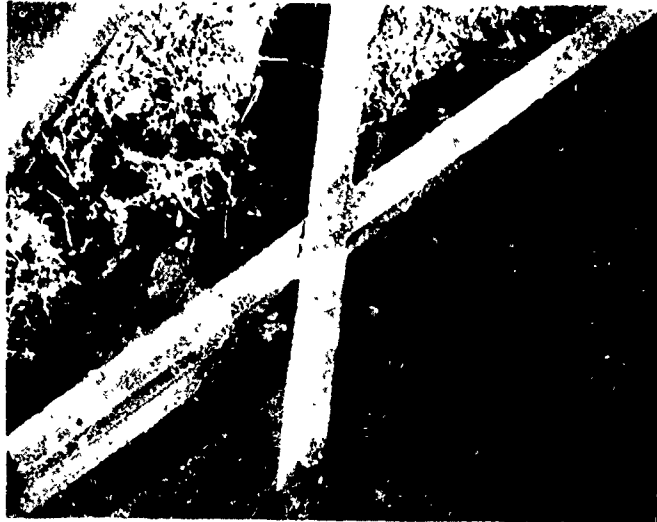
Figure I-21: Crack at "X" of Horizontal Brace.
