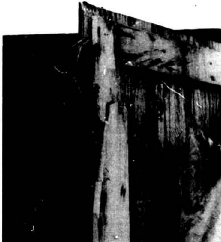
Figure 25. Interior View of Jet Forwarding Container Showing Door Damage.
