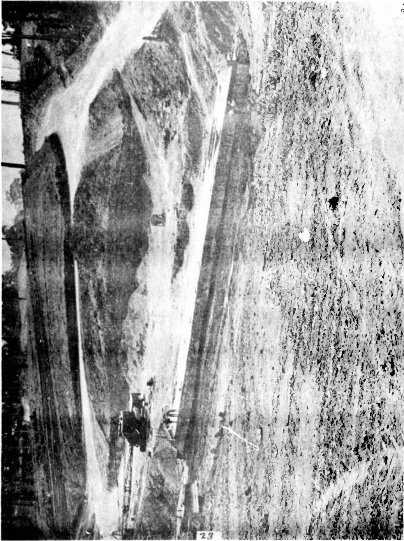
Incl #7 Double barrel 8' x 8', 53 meter reinforced concrete box culvert at K84, Rt 304.
