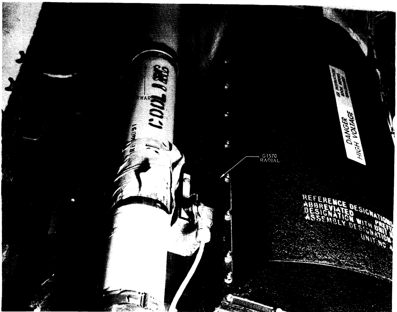
FIGURE 4.1-10 ACCELEROMETER INSTALLATION ON RATE BEACON PACKAGE
