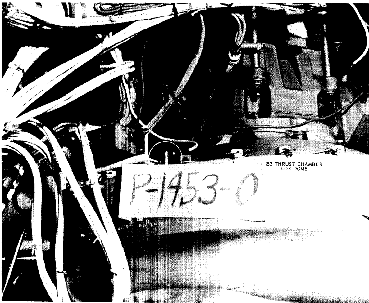
FIGURE 4.1-1 HIGH FREQUENCY ACCELEROMETER INSTALLATION
