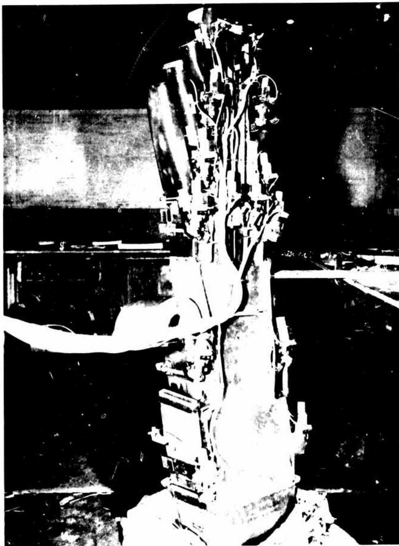
FIGURE 8.11 HIGH PRESSURE BAY VALVES (R. H.) View of Outboard Side
