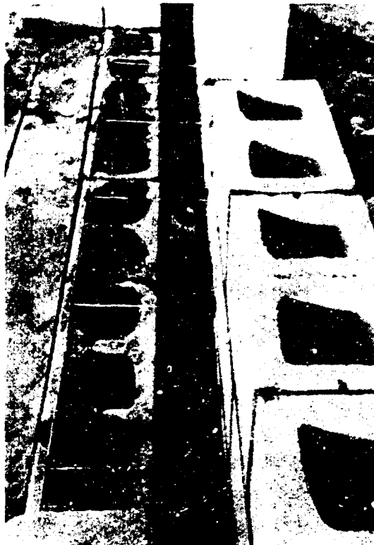
Figure 3.10 Joint reinforcement provides ties between the two wythes of the walls.
