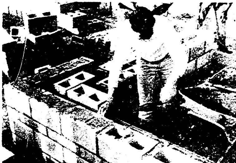
Figure 3.8 Alternate courses of 4" high solid blocks and 8" hollow core blocks were used in the outer wythe. Hollow blocks in the outer wythe were filled with mortar as each course was laid.
