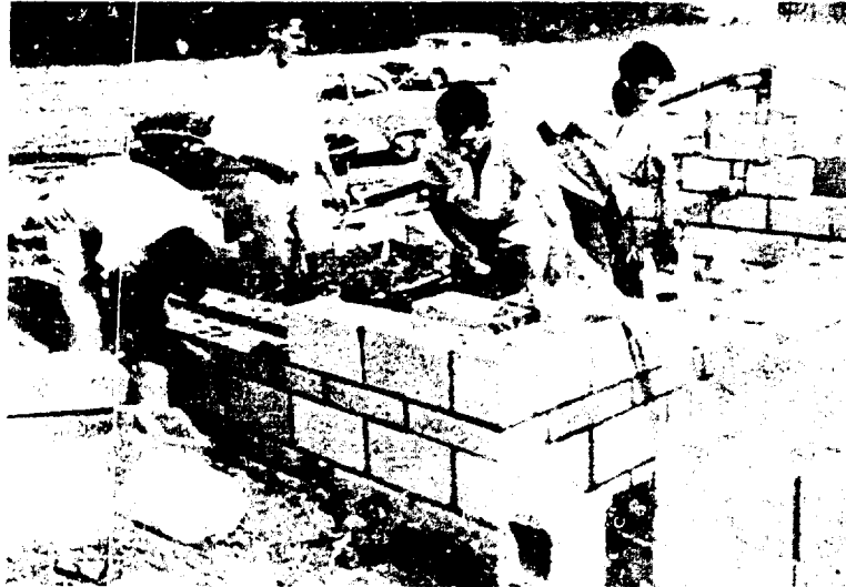
Figure 3.7 Ventilation pipes were installed in the wall cavity. Tooled joints were used on all exposed masonry walls.
