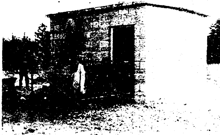
Figure 3.23 Concrete finisher applies final touches to shelter exterior.
