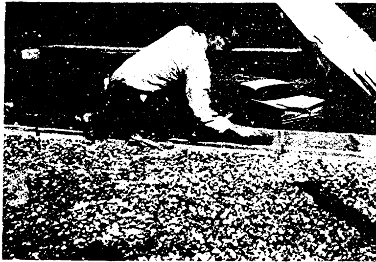
Figure 3.17 Clearing gravel from roof overhang forms. Gravel fill has been compacted and screeded to proper contour.
