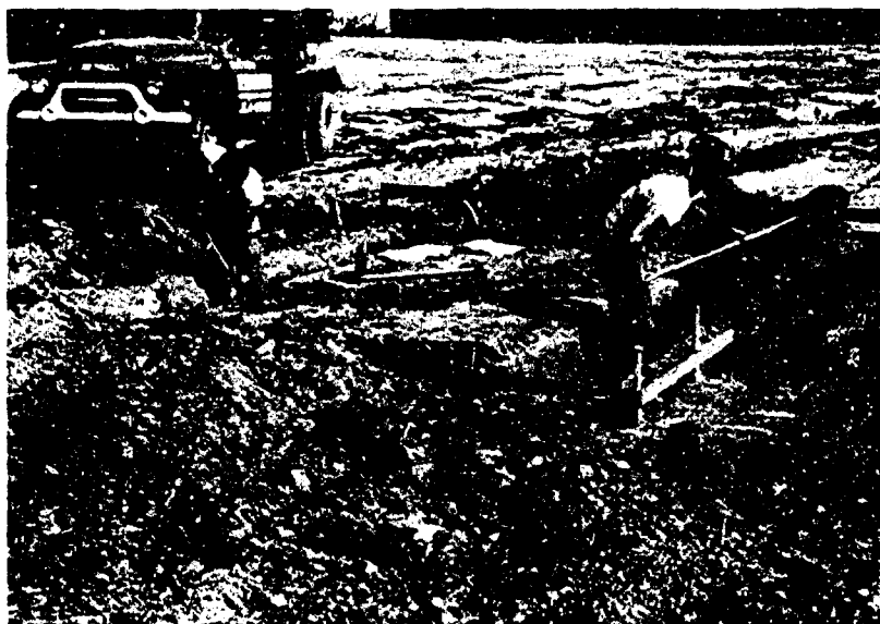
Figure 3.2 Excavation for footings was done entirely by hand using picks and shovels.
