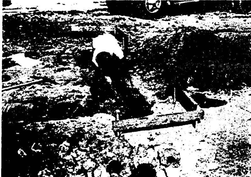
Figure 3.3 Grades for the top of footings were marked with nails driven into the side of the excavation. No forms were required for footings.
