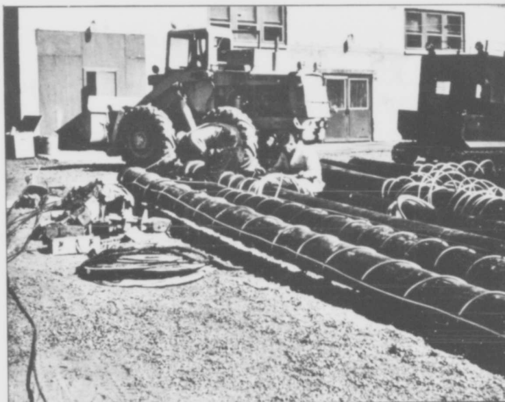
Figure 7. Refrigeration coils on timber piles for artificial freezeback.
