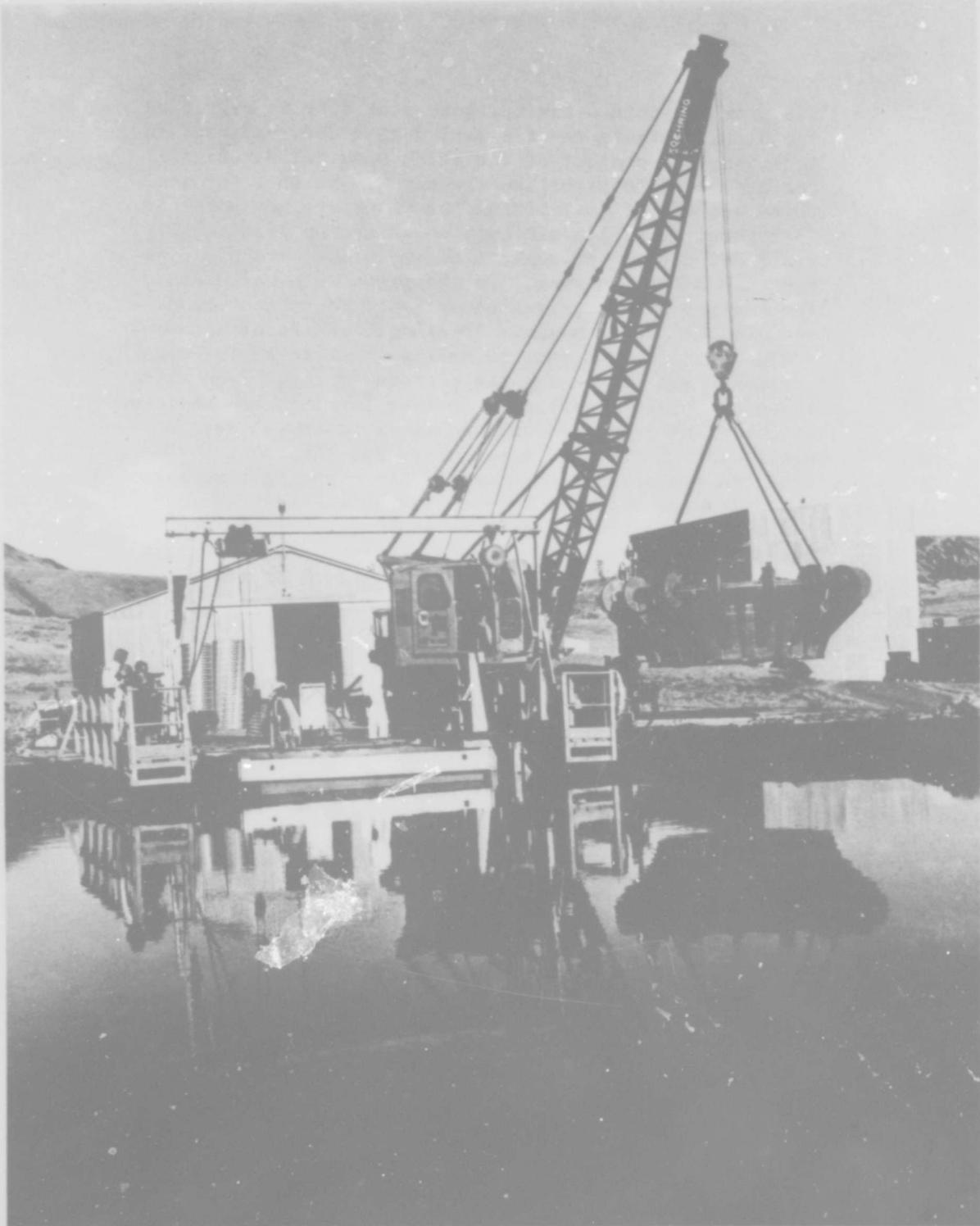
Figure 39 Lifting of 120-inch Diameter Free Forming Tool for Explosive Forming.
