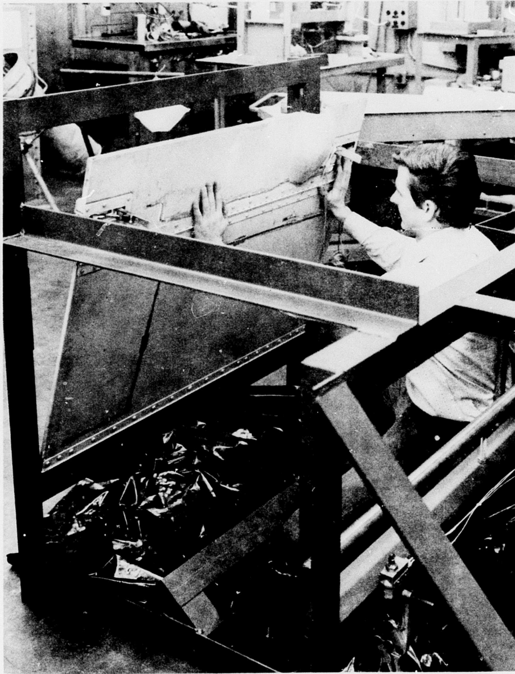
Figure 41. Work Platform Assembly, Manual Cycling.
