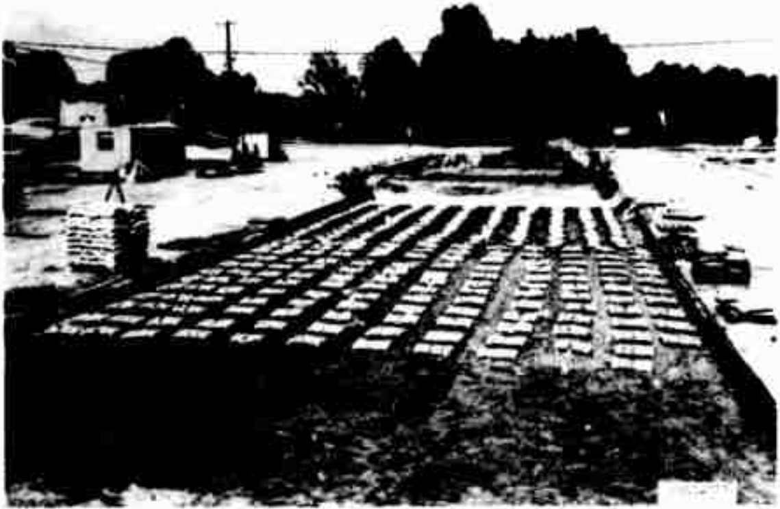
Figure 36. Bags of cement and fly ash distributed over the surface of the subgrade of items 1 and 2 of the flexible pavement test section
