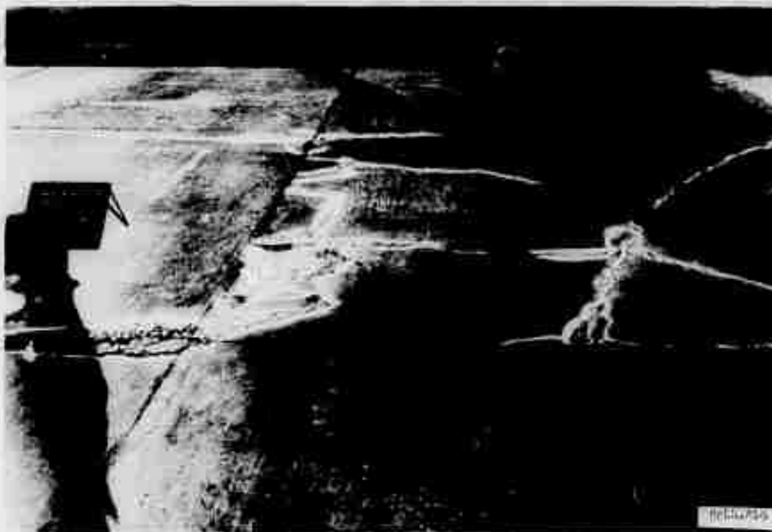
Figure A28. Subitem 5c, lane 1, rigid pavement test section, after 1230 coverages by 200-kip twin-tandem assembly
