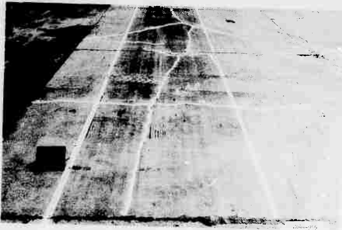
Figure A45. Item 4, lane 2, rigid pavement test section, after 200 coverages by 240-kip twin-tandem assembly
