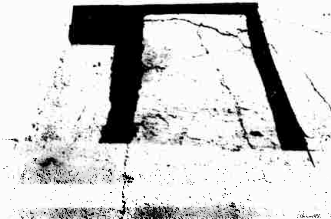
Figure B80. Cracks in lightweight concrete in subitems 4d and 5a, lane 3, flexible pavement test section, after 170 coverages of 50-kip load
