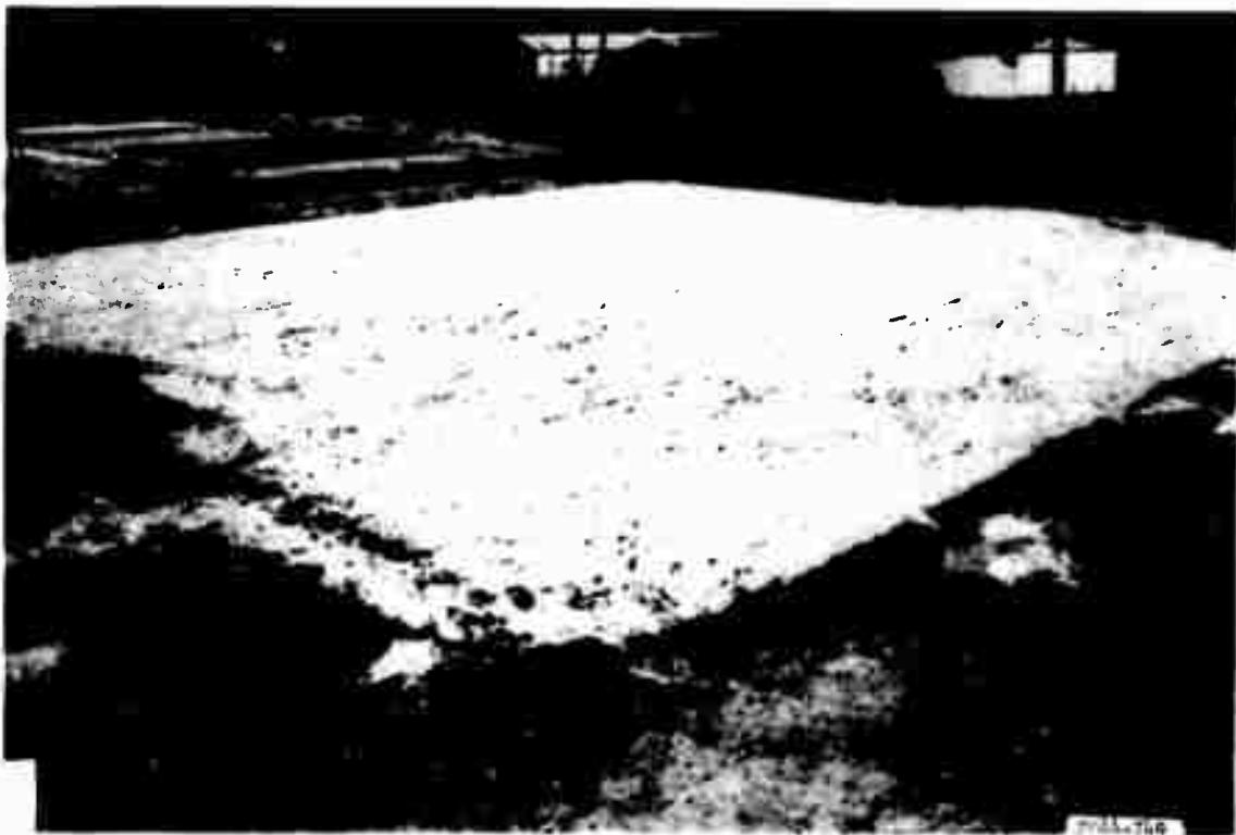
Figure 21. Completed MESL base course in item 1 of the rigid pavement test section
