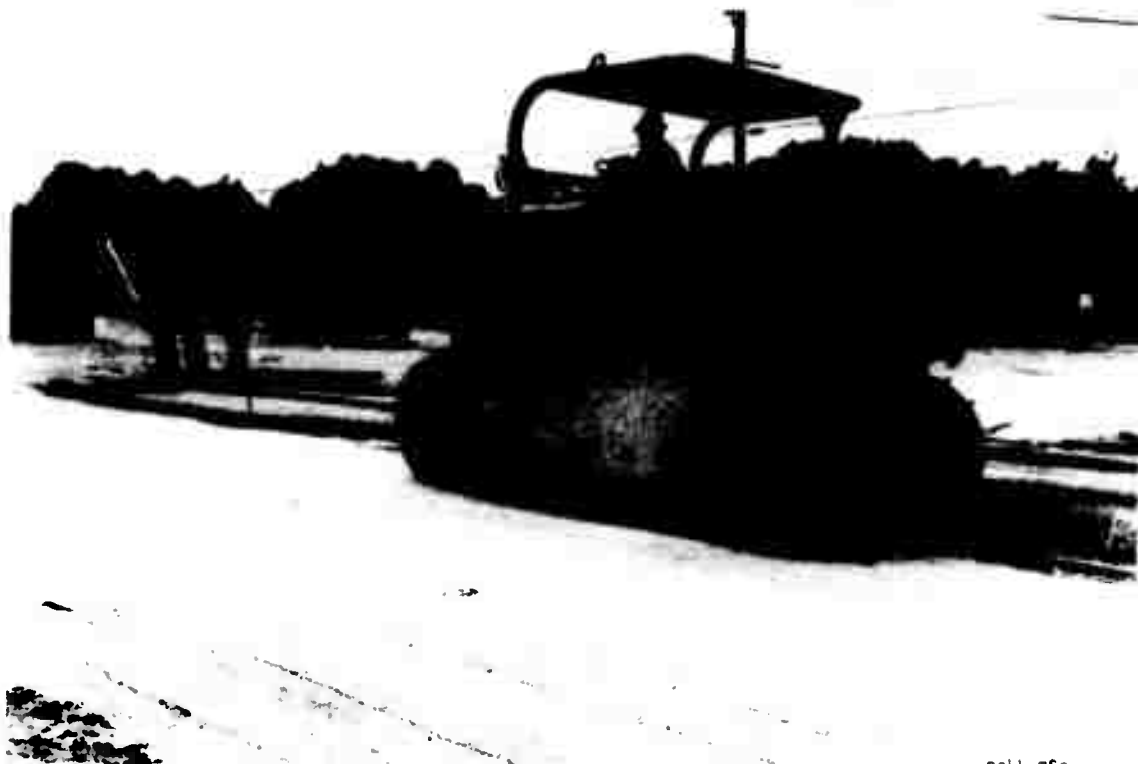
Figure 24. Compaction with the 30-ton self-propelled pneumatic-tired roller
