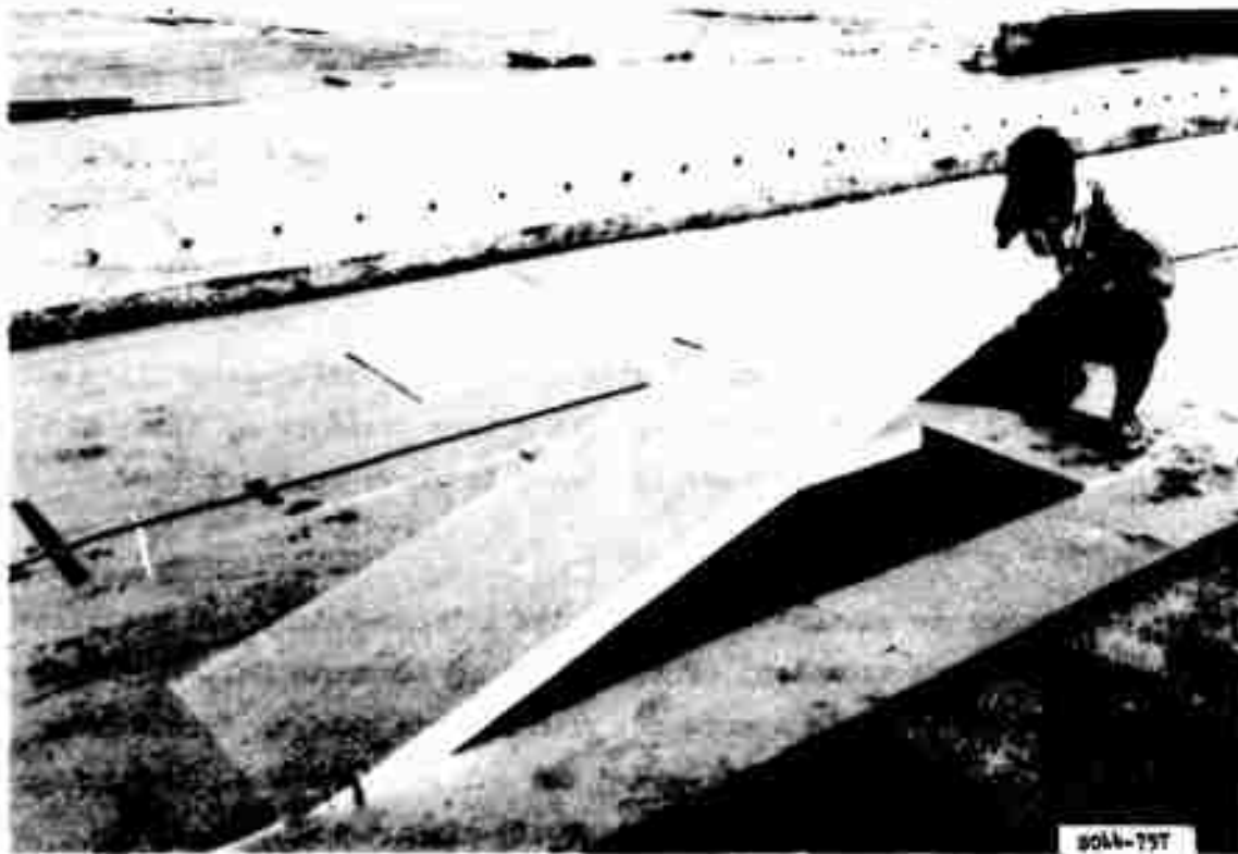
Figure 28. Polystyrene panels in place on the subgrade of item 5 of the rigid pavement test section
