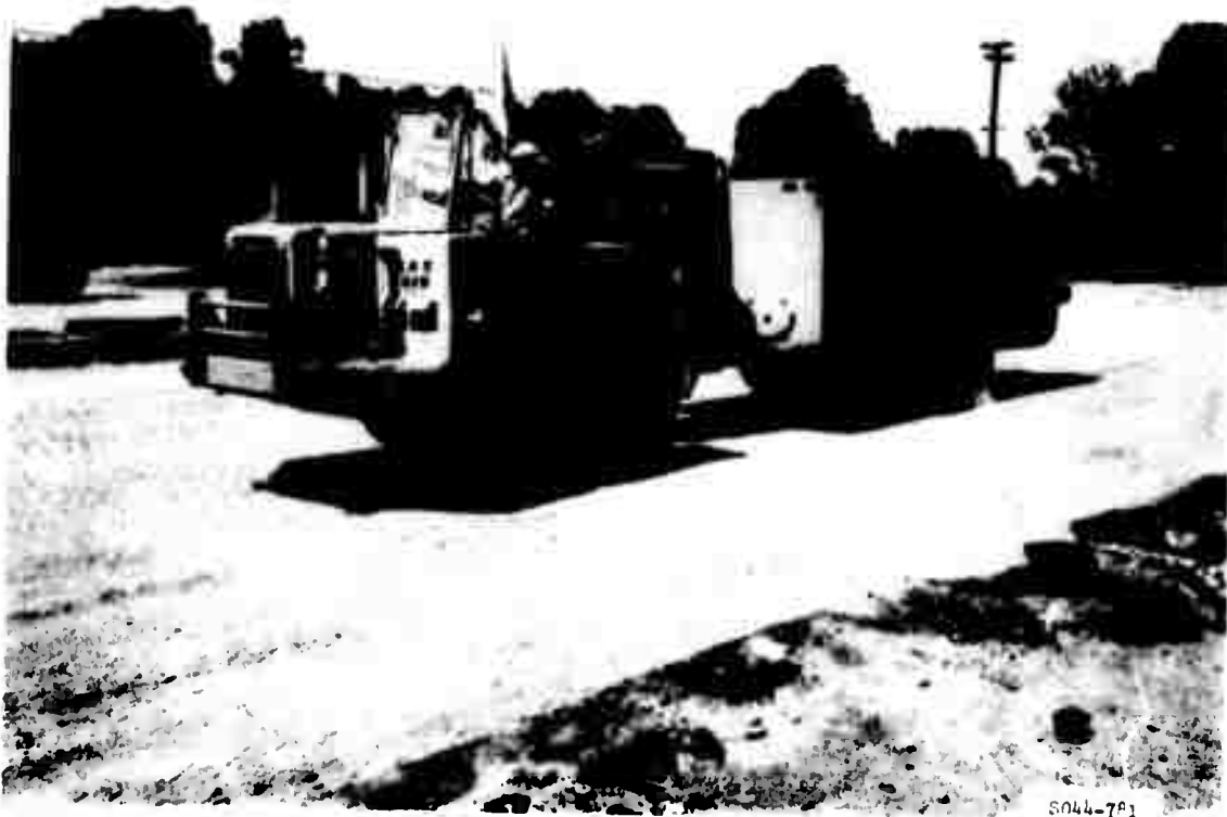
Figure 25. Compaction with the 50-ton pneumatic-tired roller
