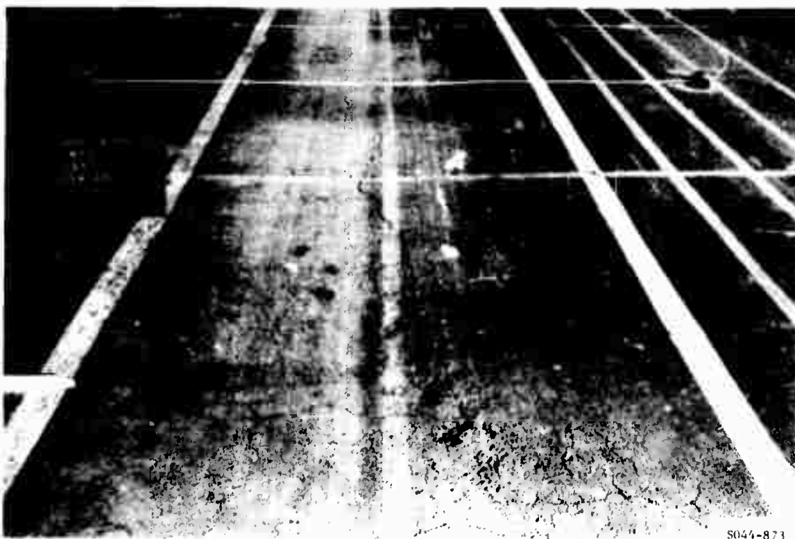
Figure B54. Cracking and deformation in subitem 4b, lane 3, flexible pavement test section, at failure after 170 coverages of 50-kip single-wheel assembly
