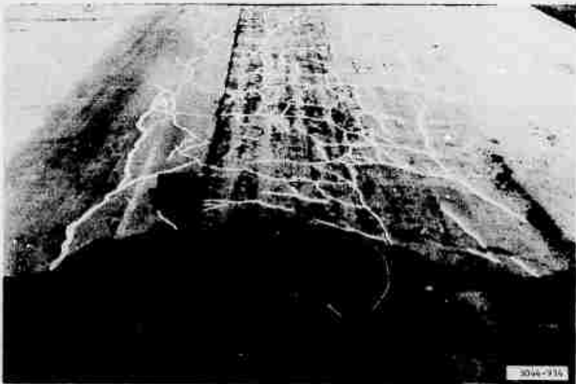
Figure A4. Item 1, lane 1, rigid pavement test section, after 3000 coverages by 200-kip twin-tandem assembly
