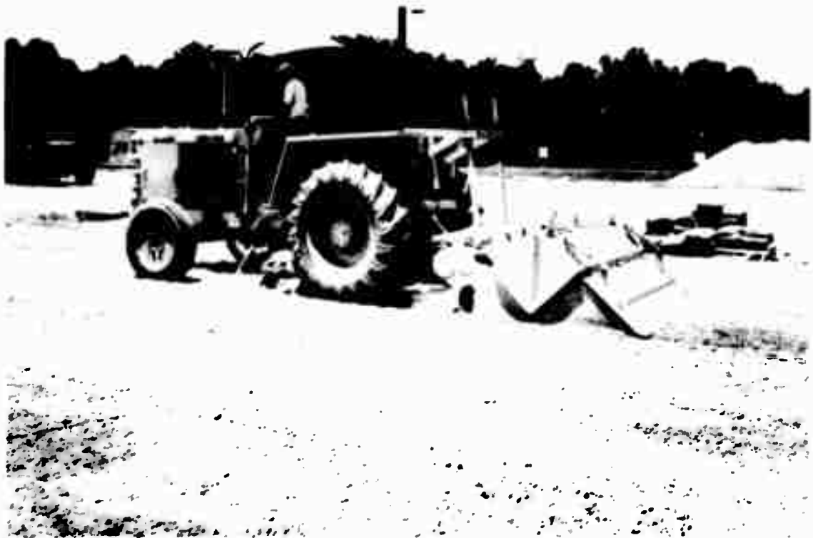
Figure 37. In-place mixing of treated soil with pulvimixer
