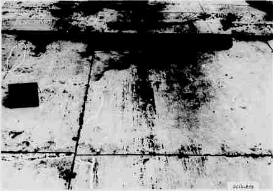
Figure A25. Subitem 5b, lane 1, rigid pavement test section, after 1770 coverages by 200-kip twin-tandem assembly
