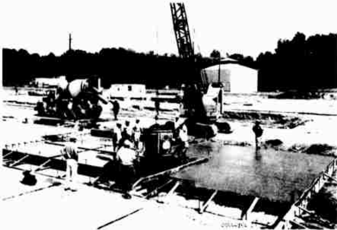
Figure 33. Placement of concrete over insulating materials in item 5 of the rigid pavement test section
