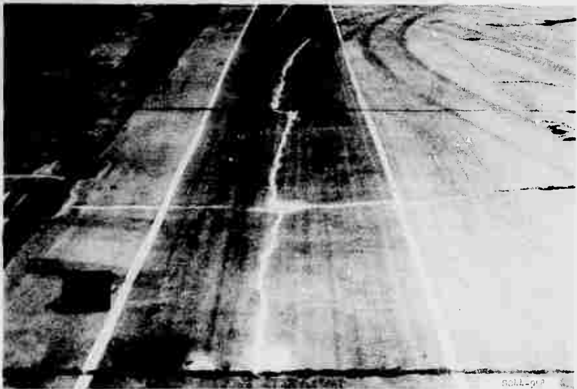
Figure A41. Item 3, lane 2, rigid pavement test section, after 200 coverages by 240-kip twin-tandem assembly
