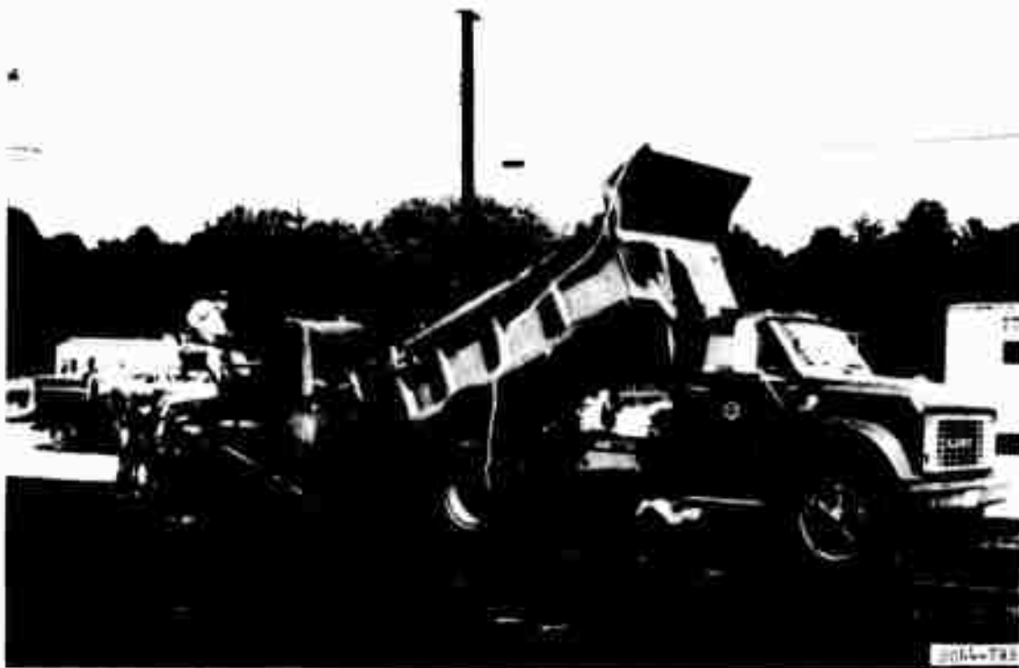
Figure 4C. Placement of 3-in.-thick asphaltic concrete surface course on the flexible pavement test section
