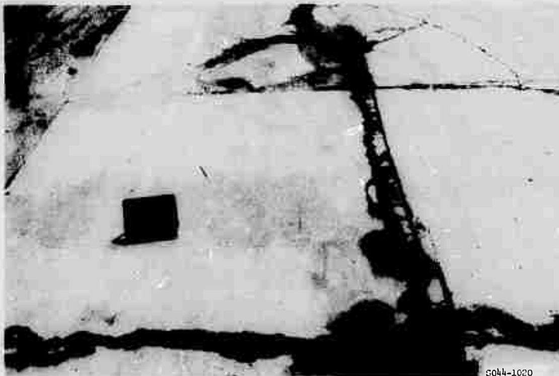
Figure A54. Subitem 5c, lane 2, rigid pavement test section, after 840 coverages by 240-kip twin-tandem assembly
