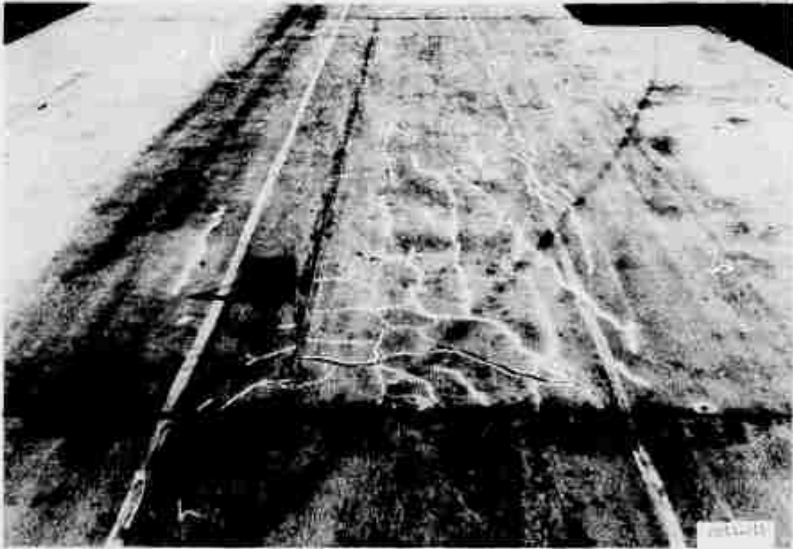
Figure A9. Item 2, lane 1, rigid pavement test section, after 1000 coverages by 200-kip twin-tandem assembly
