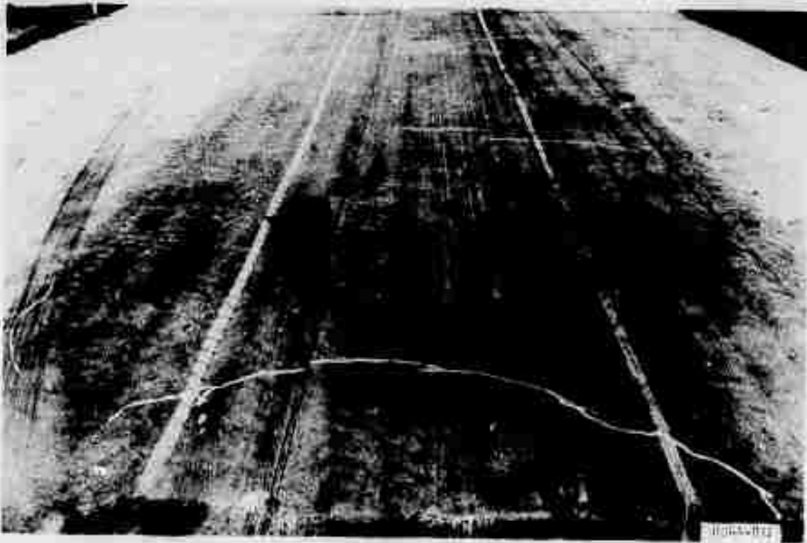
Figure A2. Item 1, lane 1, rigid pavement test section, after 200 coverages by 200-kip twin-tandem assembly
