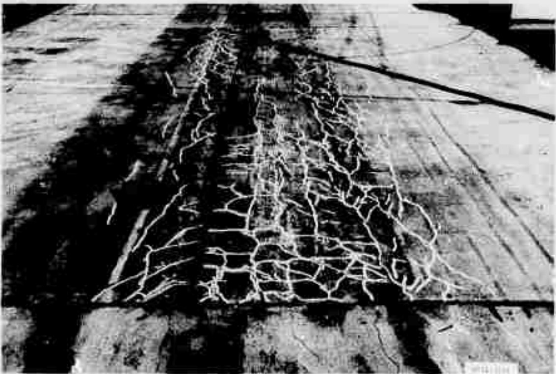
Figure A10. Item 2, lane 1, rigid pavement test section, after 1770 coverages by 200-kip twin-tandem assembly
