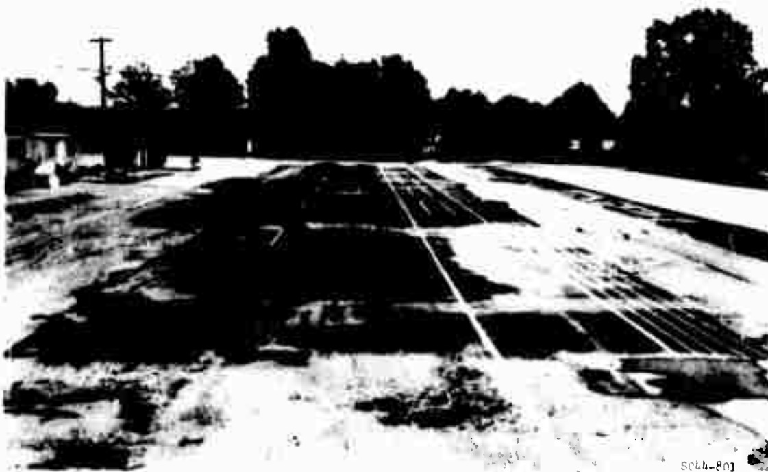
Figure 41. Overall view of completed flexible pavement test section
