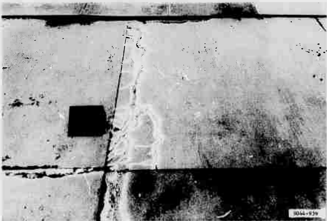
Figure A26. Subitem 5b, lane 1, rigid pavement test section, after 3000 coverages by 200-kip twin-tandem assembly
