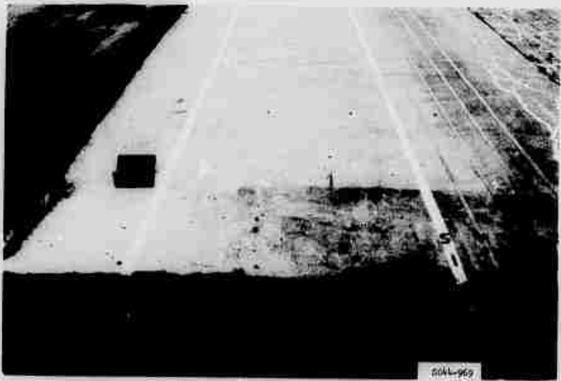
Figure A31. Item 1, lane 2, rigid pavement test section, prior to traffic
