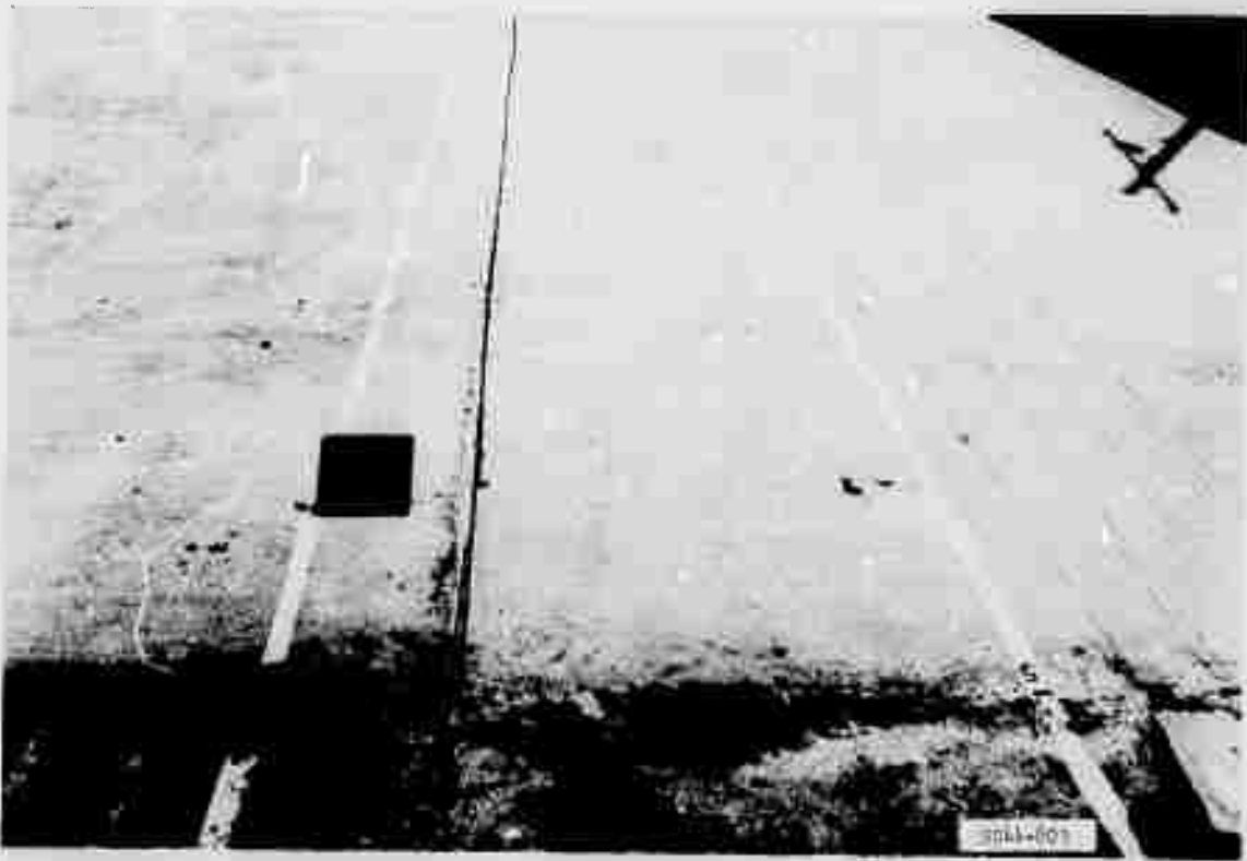
Figure A1. Item 1, lane 1, rigid pavement test section, prior to traffic
