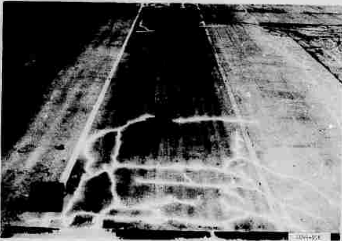
Figure A33. Item 1, lane 2, rigid pavement test section, after 200 coverages by 240-kip twin-tandem assembly
