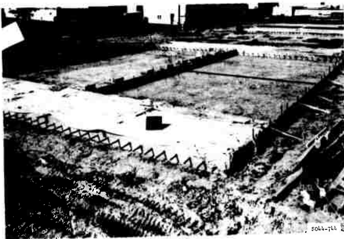
Figure 31. Transition slabs in place between the rigid pavement test items
