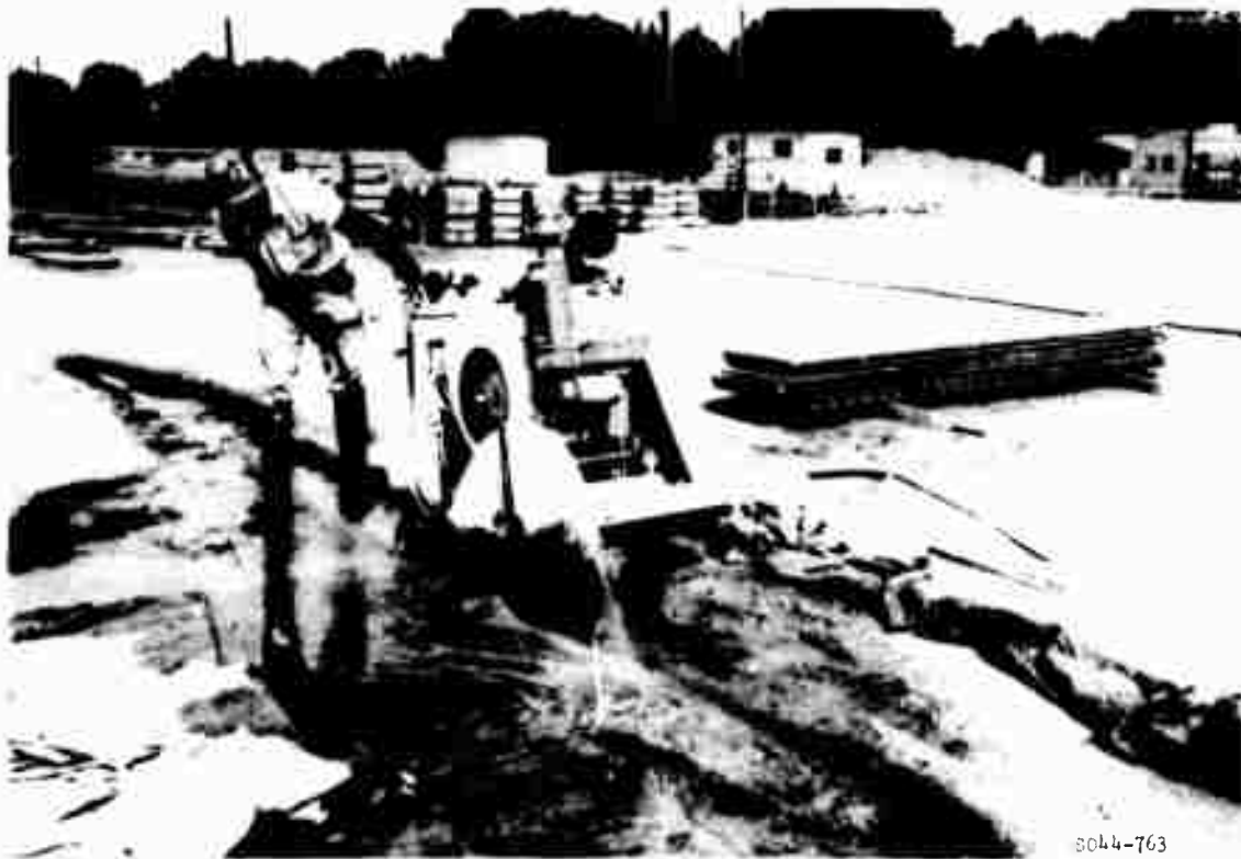
Figure 34. Joint sawing operations in the rigid pavement test section
