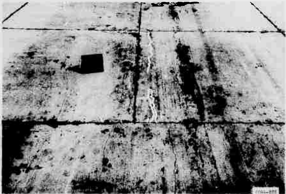
Figure A22. Subitem 5a, lane 1, rigid pavement test section, after 1770 coverages by 200-kip twin-tandem assembly
