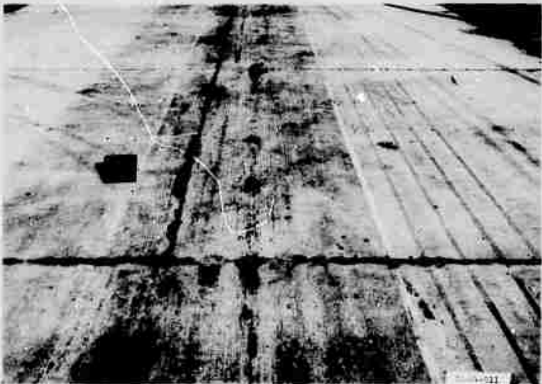
Figure A18. Item 4, lane 1, rigid pavement test section, after 1770 coverages by 200-kip twin-tandem assembly
