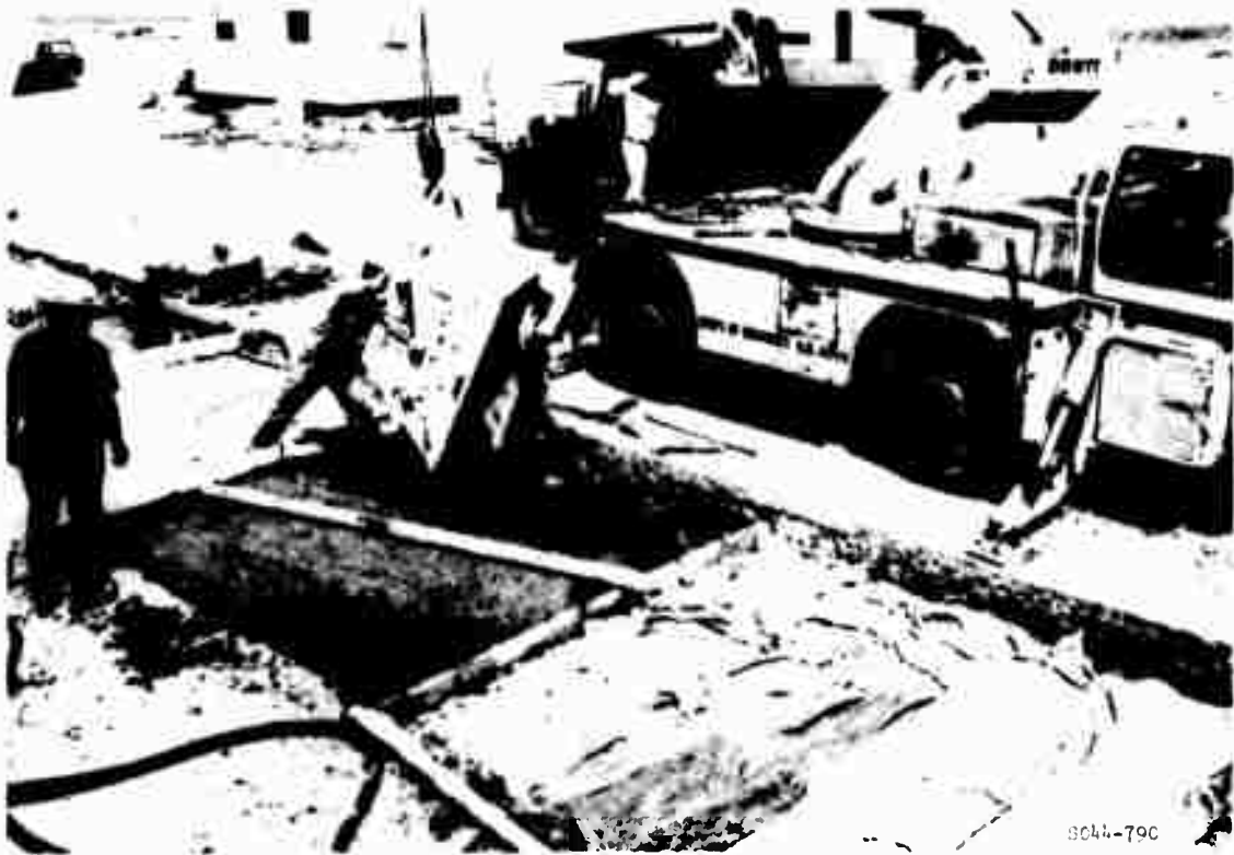
Figure 38. Placement of lightweight concrete insulating materials in item 5 of the flexible pavement test section
