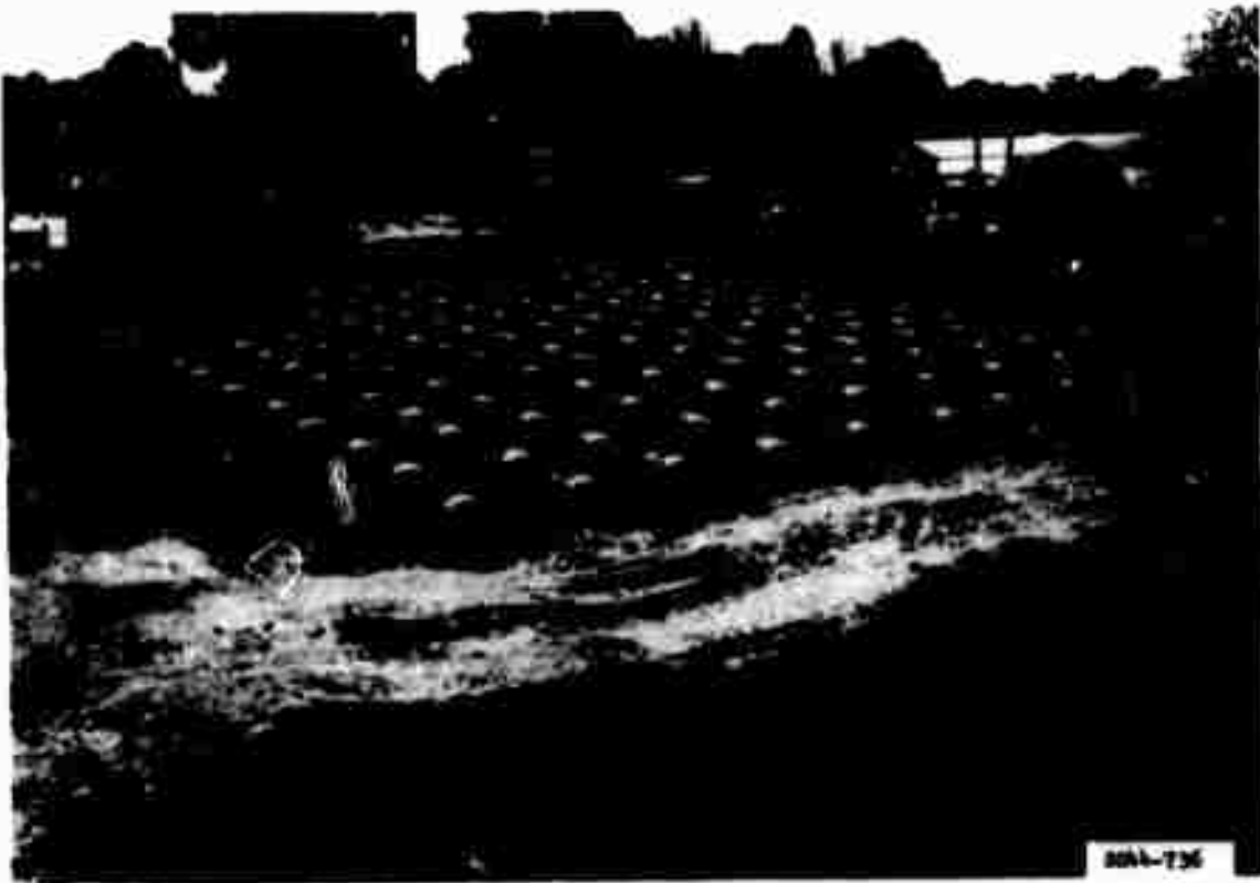
Figure 22. Bags of cement distributed over the surface of the base of item 2 of the rigid pavement test section
