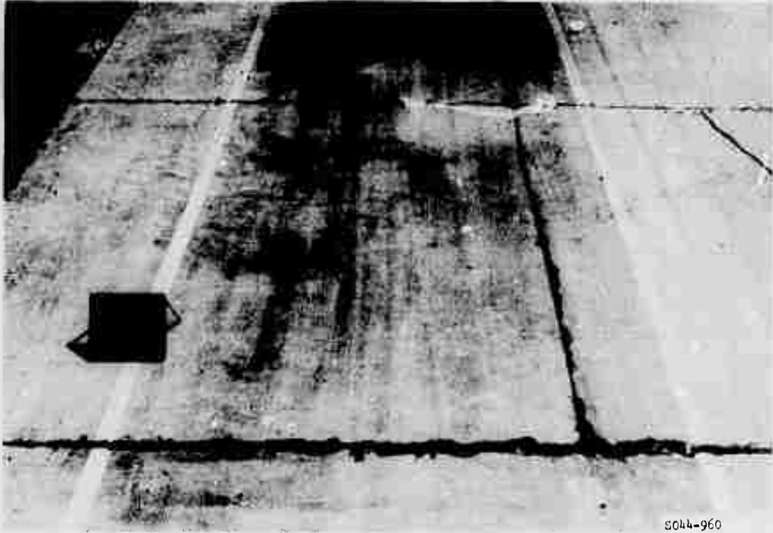
Figure A48. Subitem 5a, lane 2, rigid pavement test section, after 200 coverages by 240-kip twin-tandem assembly
