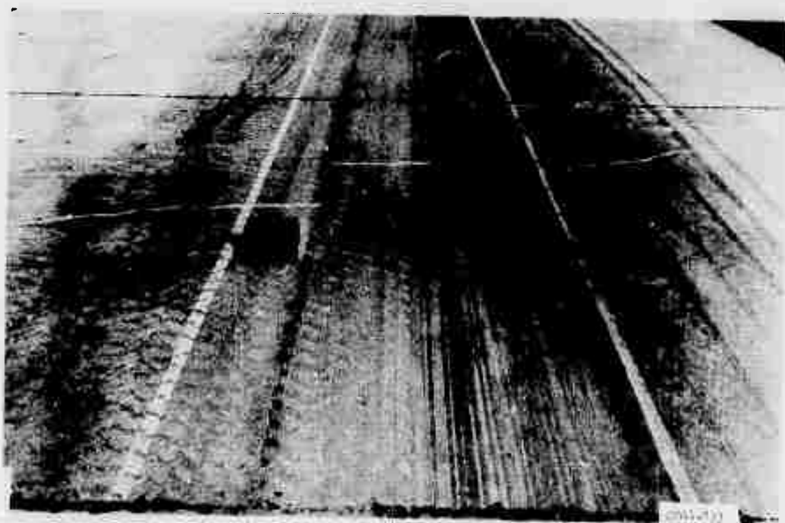
Figure A13. Item 3, lane 1, rigid pavement test section, after 200 coverages by 200-kip twin-tandem assembly
