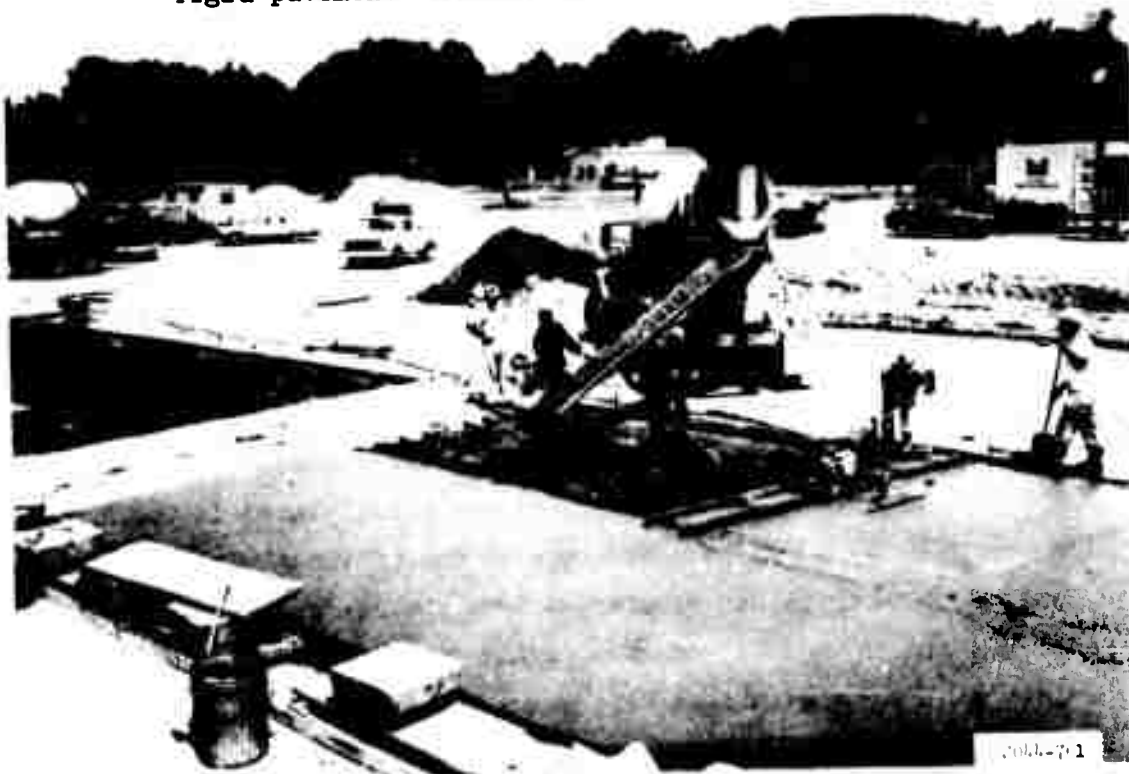
Figure 32. Placement of fibrous-reinforced concrete over insulating materials in item 2 of the rigid pavement test section
