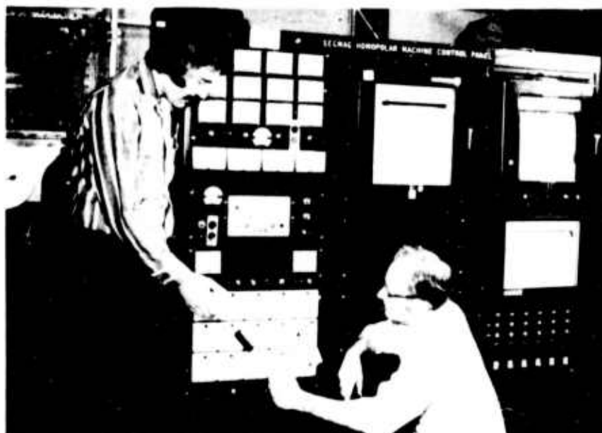
Fig. 5-7 -- Instrumentation and control panel for the SEGMAG generator test bed
