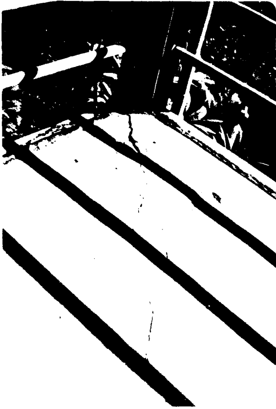
Figure 19. Second deck walkway, cable building, Midway.
