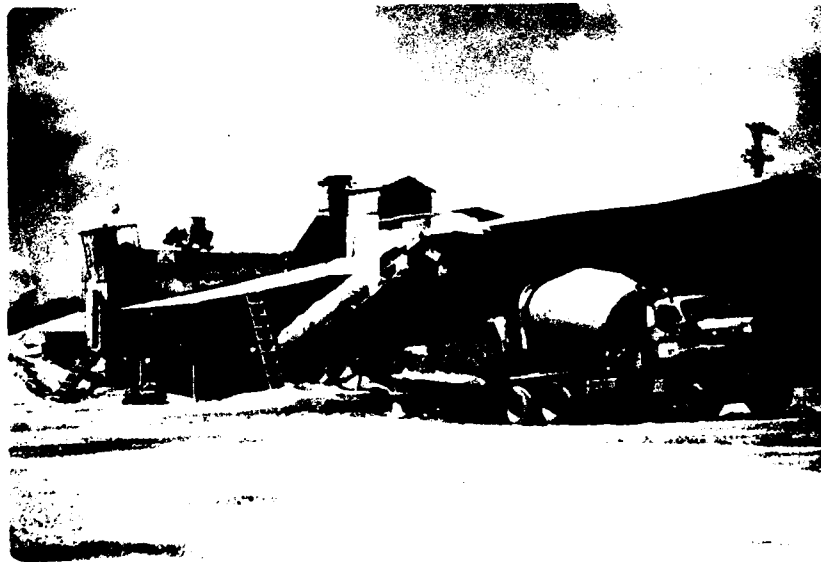
Figure 4. Concrete batch plant and transit mixer, Hyundai Quarry, Guam.
